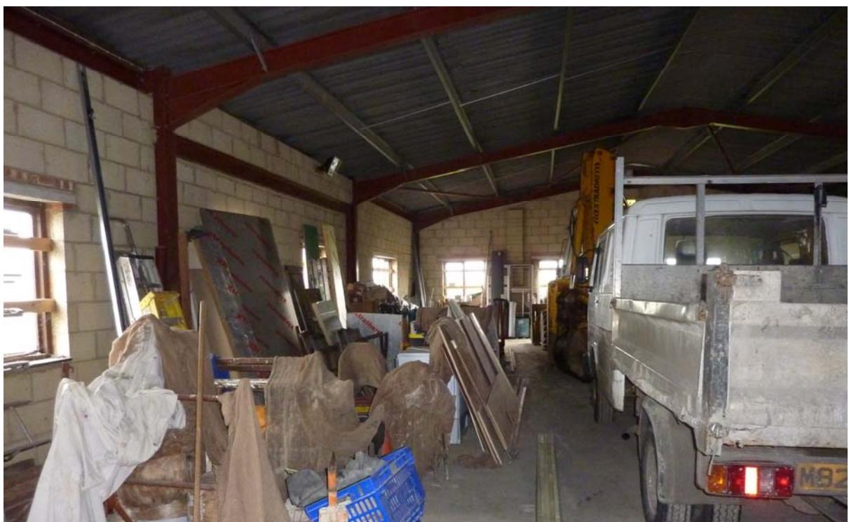
Figure 4: View inside eastern building used for general storage
