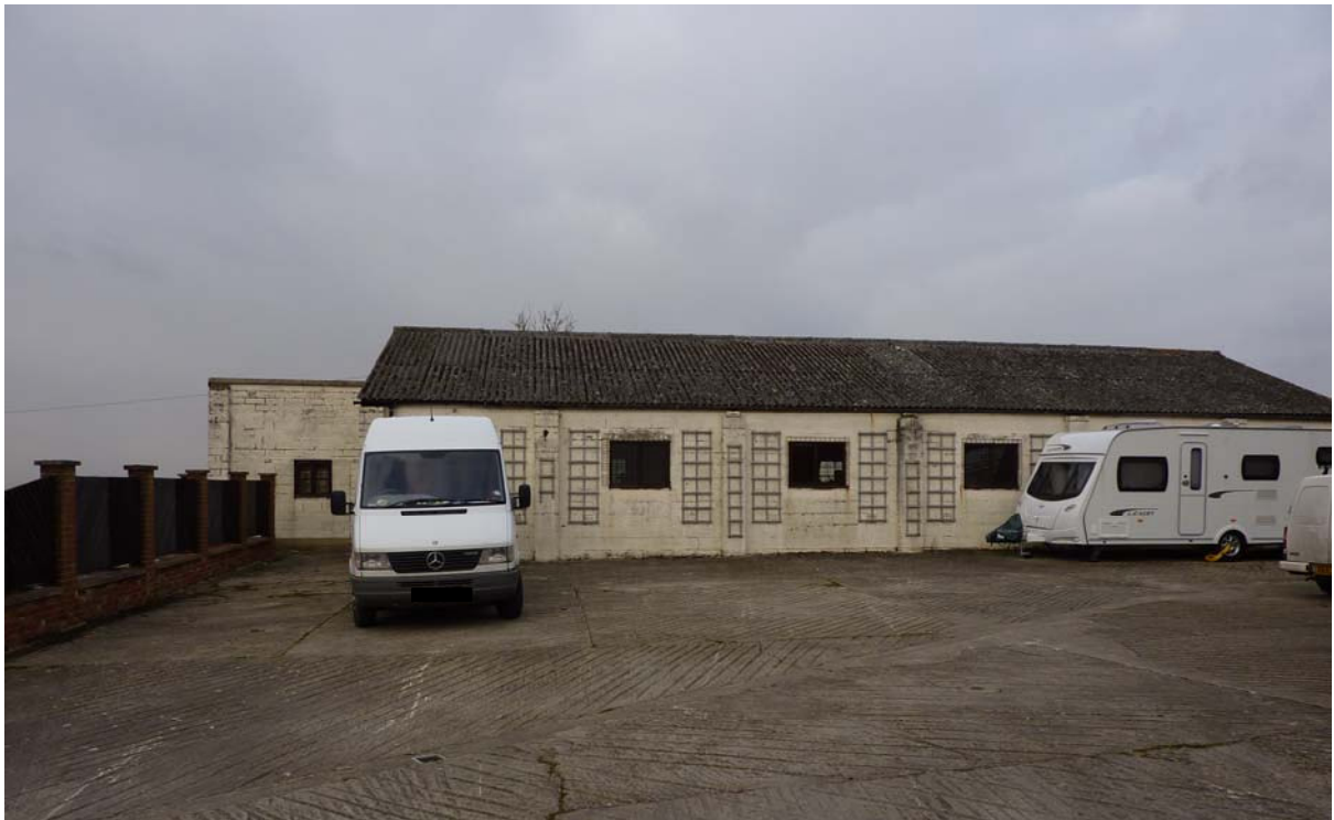
Figure 1: Western workshop used for carpentry / joinery looking north
