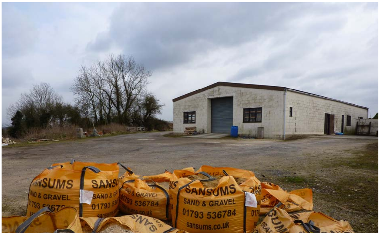
Figure 3: Eastern building used for general storage purposes looking southeast
