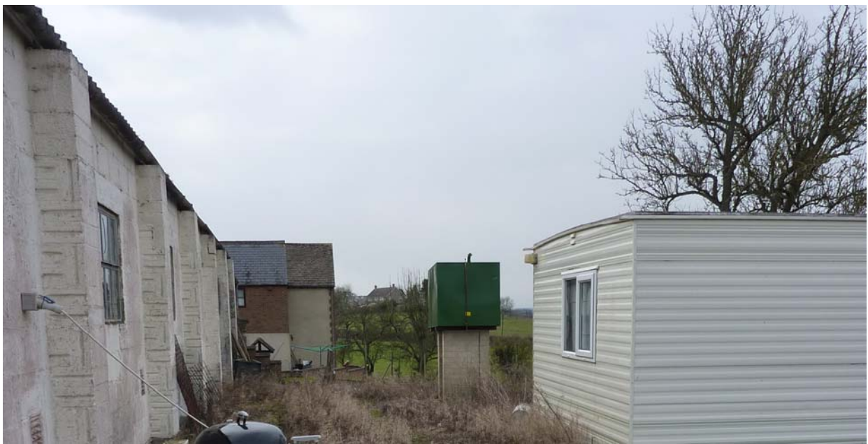
Figure 9: Above ground fuel tank
