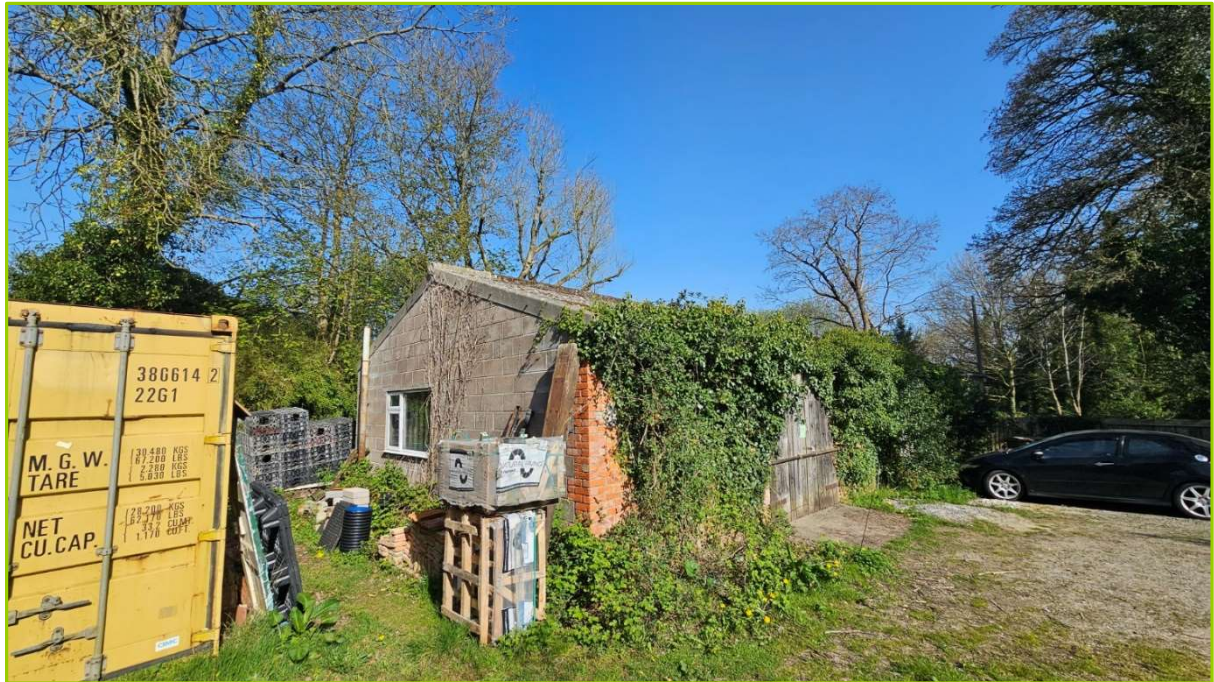
Photo 4 - View looking north showing frontage and workshop.
