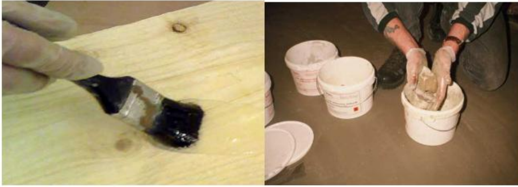
Priming wood with Epoxy Primer. Mixing Mouldable Epoxy
