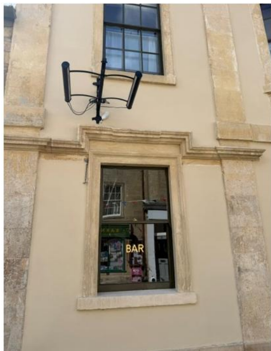
Below: Existing bracket and lighting
