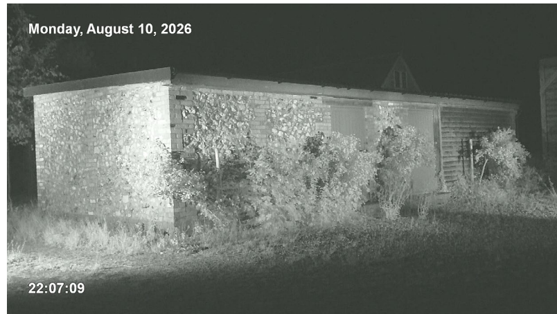
Figure 3: southwestern corner of the building
