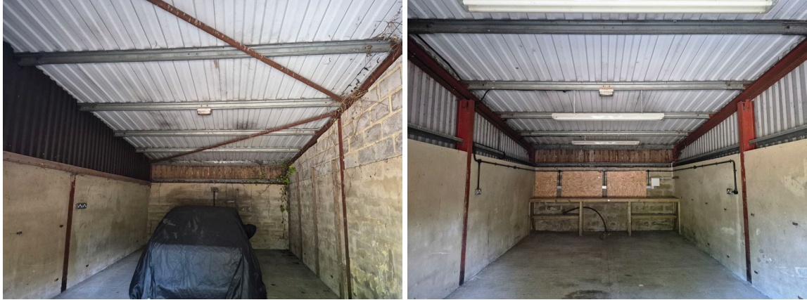
Figure 6 and 7: Southern and central rooms within B1.
