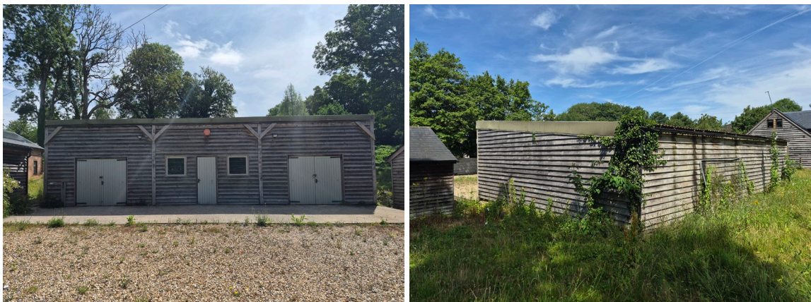
Figure 4 and 5: Western and southeastern elevations of B1.
