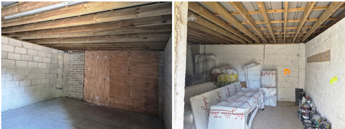
Figure 11 and 12: Eastern and western rooms within B2.
