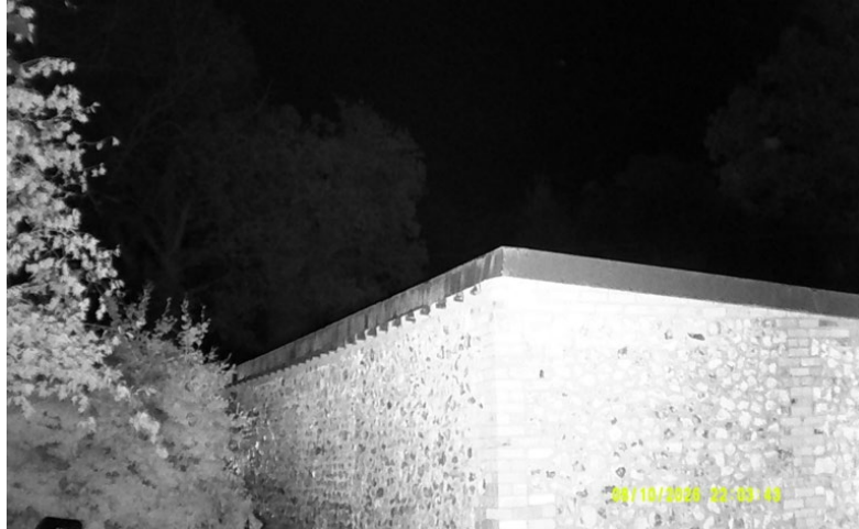
Figure 2: Northwestern corner of the building
