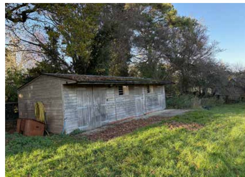
The existing building
