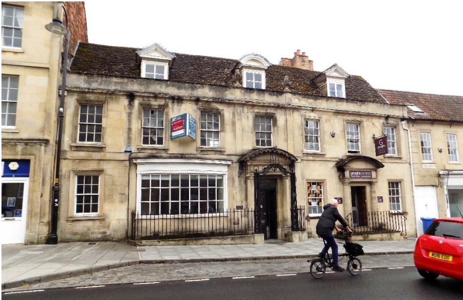
Fig.10: View of the north elevation of Nos 2 and 3 Fore Street, showing the twentieth-century dormers, left-hand ground floor window (former doorway to passage), bay window in reformed opening, cast iron panelled standards with a lamp overthrow and the wholly new ground-floor facade and door surround to No.2.
