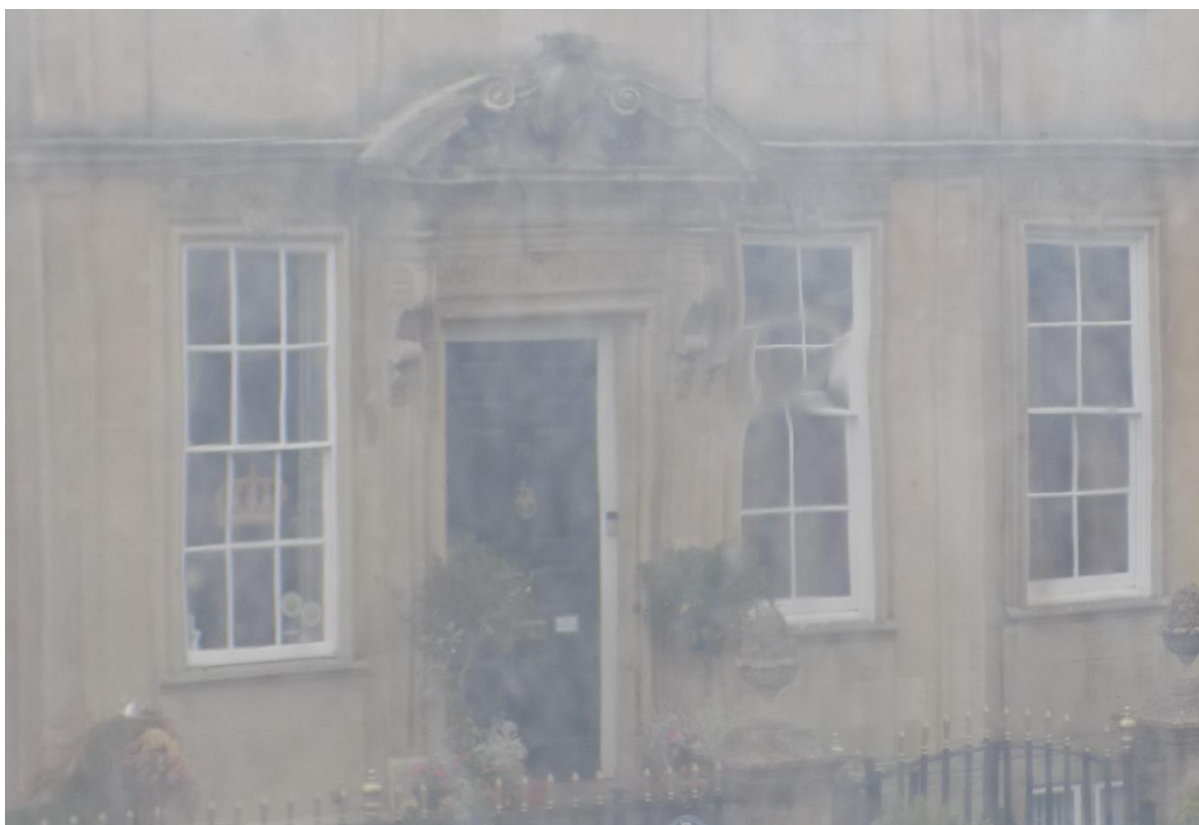
Fig.35: Detail of view through front-facing pane, showing optical deformation typical of hand-made glass.
