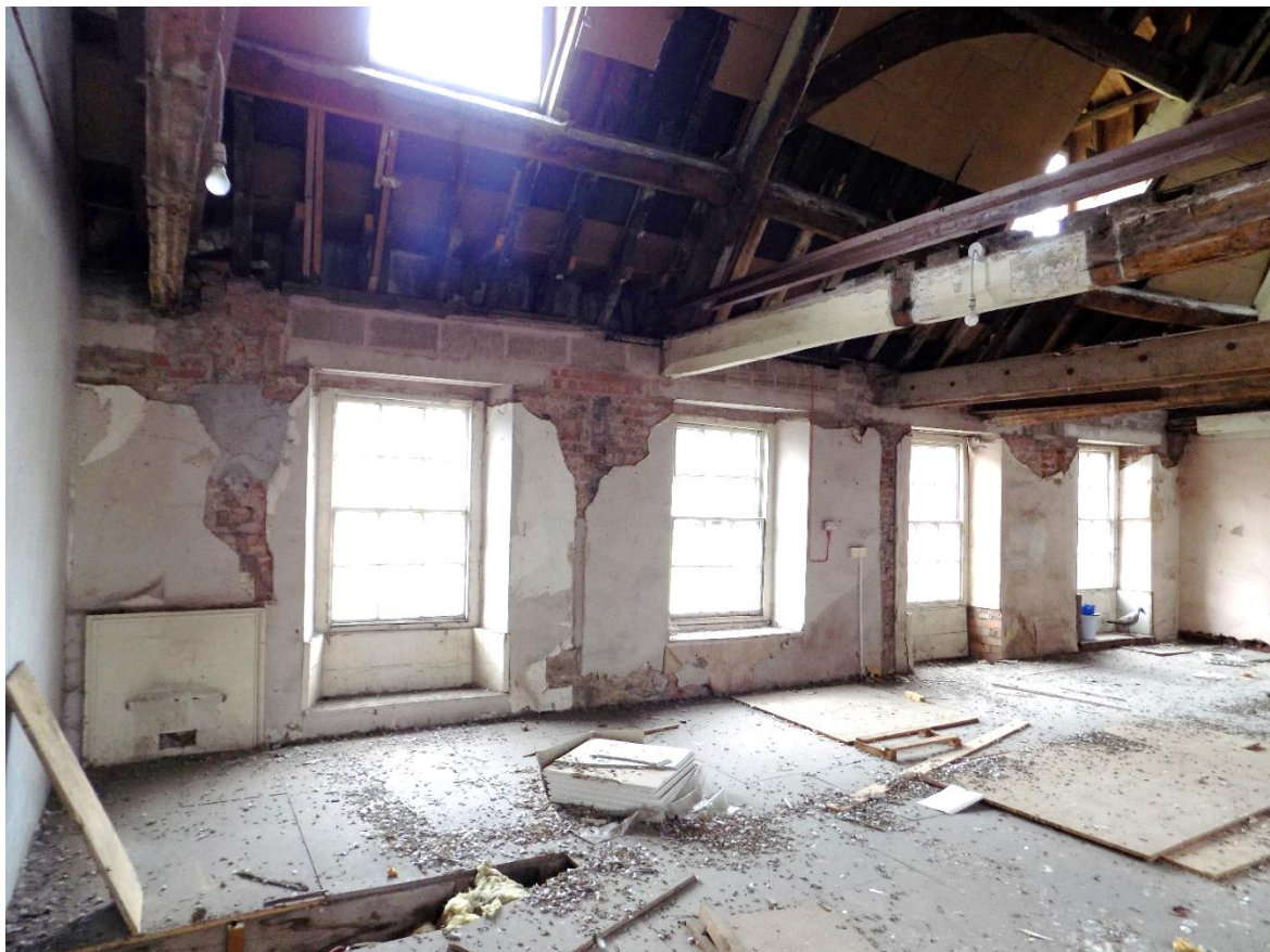
Fig.21: General view of the first floor, looking north-east, showing modern false floor.
