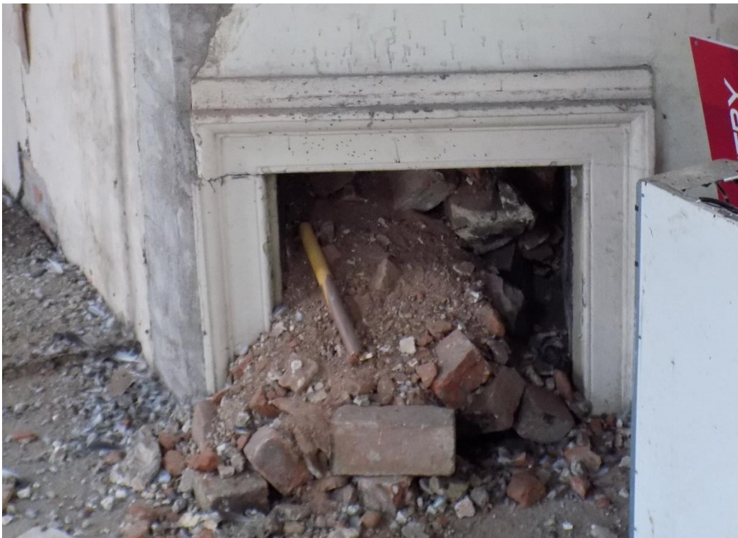
Fig.23: Detail of suspected fireplace, showing ovolo mouldings.
