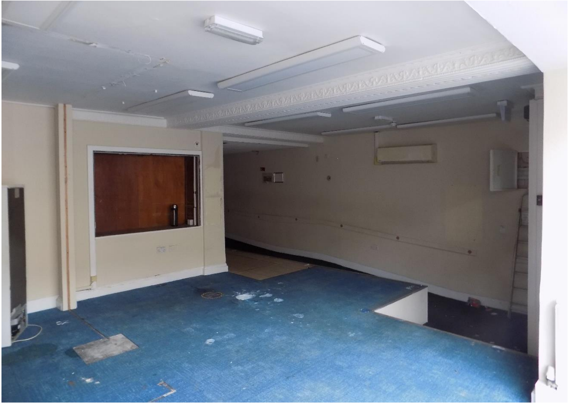
Fig.16: Ground-floor internal view, frontage range, showing moulded beam and raised floor.
