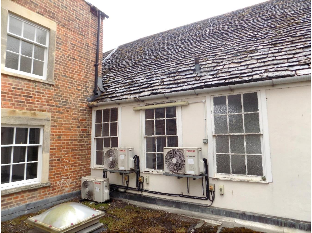
Fig.14: Rear detail, showing sash windows with no horns set flush with the outer face, indicating a likely pre-1850 date. The sills and architraves are modern.
