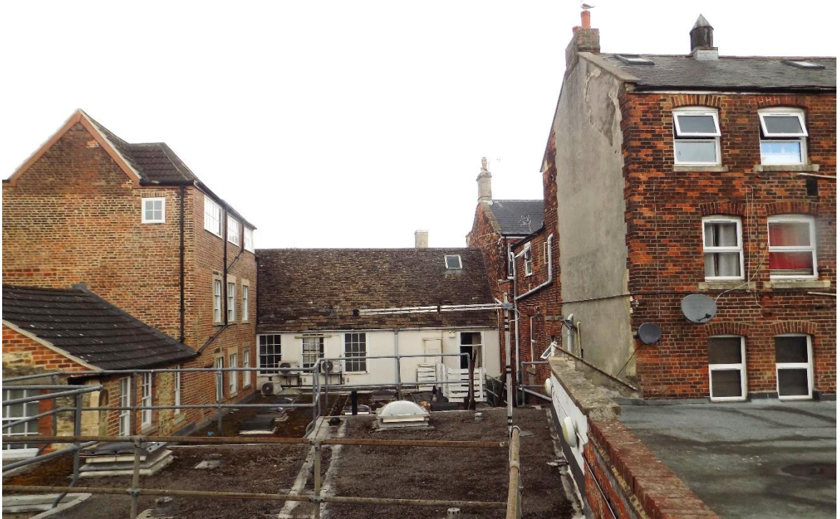
Fig.12: Rear view of No.3 Fore Street as seen from the flat roof of the rear extension, showing four-storey buildings to either side.
