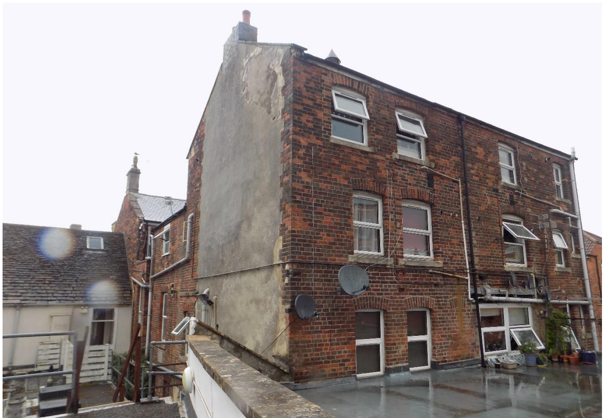
Fig.50: View looking north-east from the location of the proposed four-storey block, showing the four-storey back range of No.4 Fore Street.
