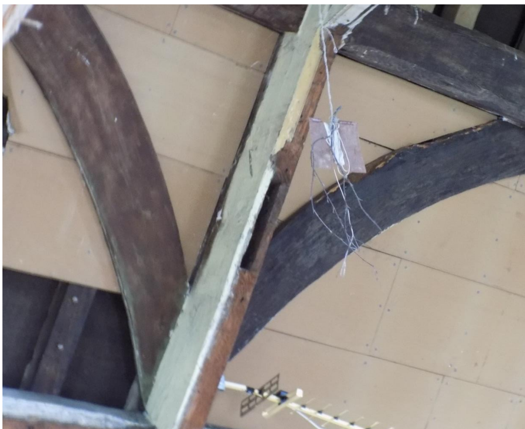
Fig.43: Detail of curved wind-braces and empty mortice for queen posts.
