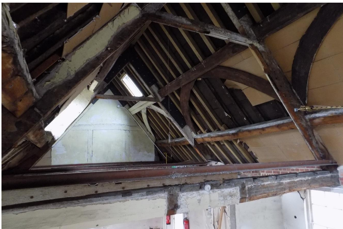
Fig.39: Attic view looking east, showing second tie from east notched for joists at northern end only of eastern face.
