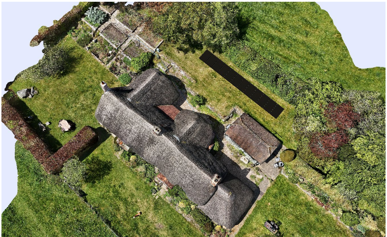
Aerial view of the property and its curtilage, illustrating the relationship between the listed cottage, outbuildings, rear garden and the proposed location of the ground-mounted solar array.
