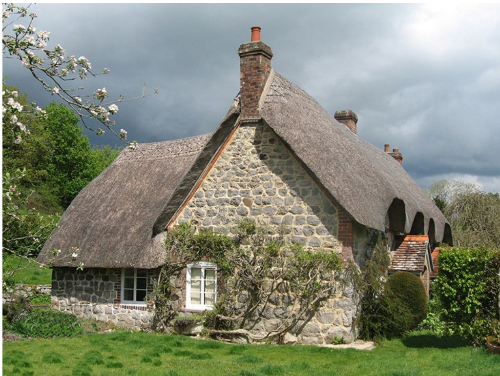
The south-west elevation illustrates the traditional gable end constructed in sarsen stone with the thatched roof extending over the historic single-storey form and later side extension.
