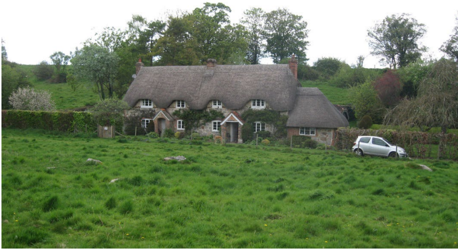
Main southeast elevation, viewed from the adjacent pasture, showing the long straw thatched roof, eyebrow dormers and traditional stone, brick and rendered walls.
