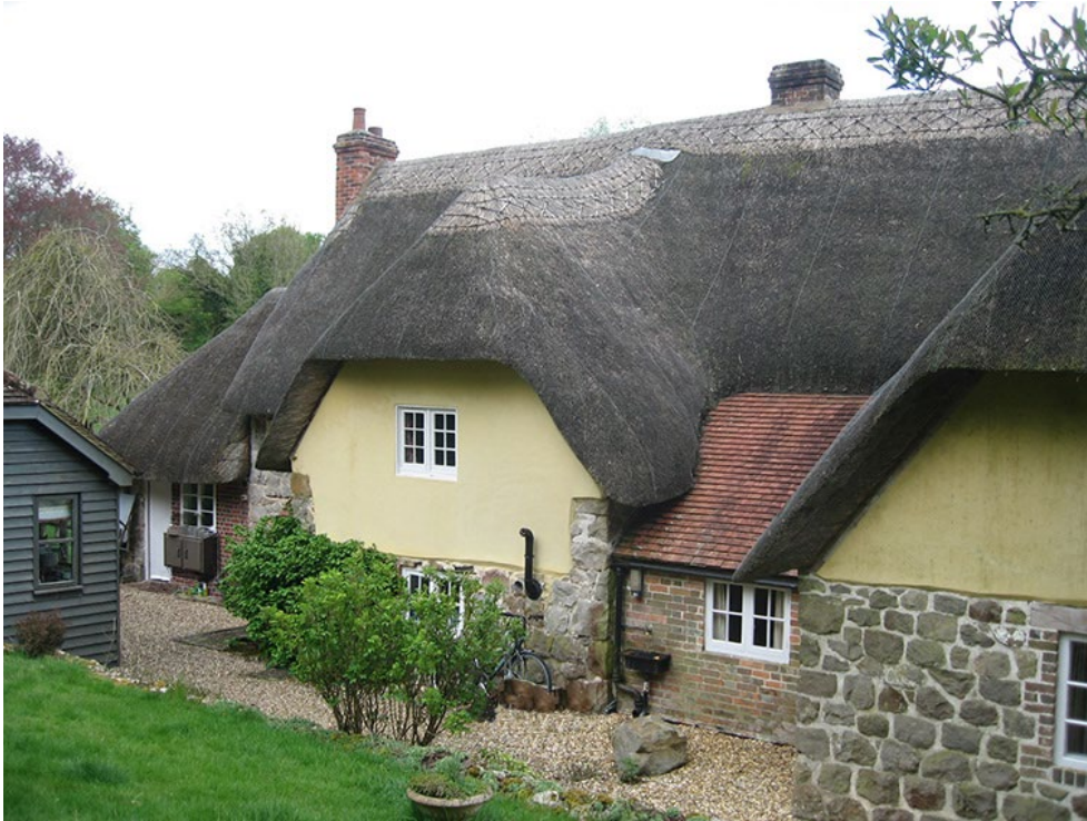
The rear elevation shows the historic extensions and lean-to additions, together with the varied use of render, brick and sarsen stone characteristic of the building's evolution.
