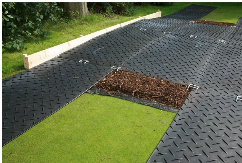
Figure F: An example of load-spreading boards and woodchip mulch used as ground protection.
