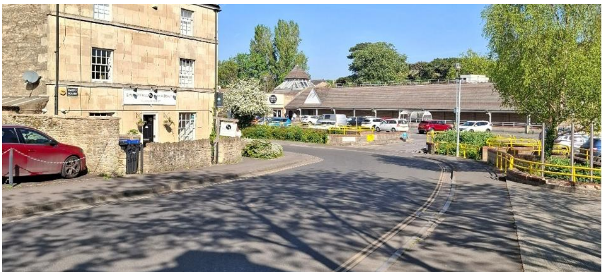
Figure 7: View from Emery Lane of the former Tesco supermarket building and car park.
