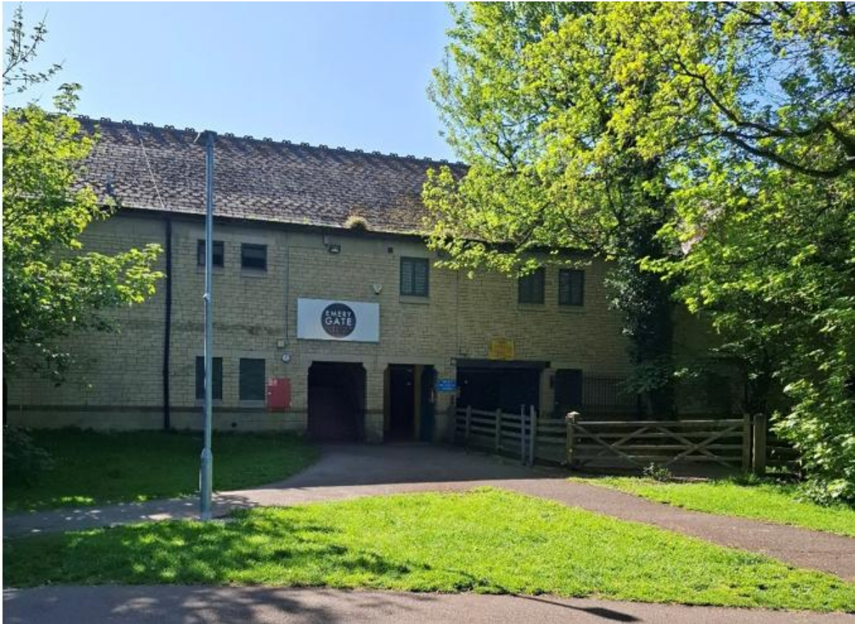
Figure 6: View from Island Park of the existing built form. Existing pedestrian access to Emery Gate Shopping Centre via stairs to the left, pedestrian access to the car park in the centre and vehicular access to the right of the image.
