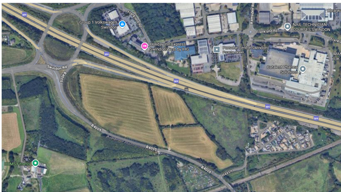
Figure 2: Aerial Image of the site taken from Google maps
