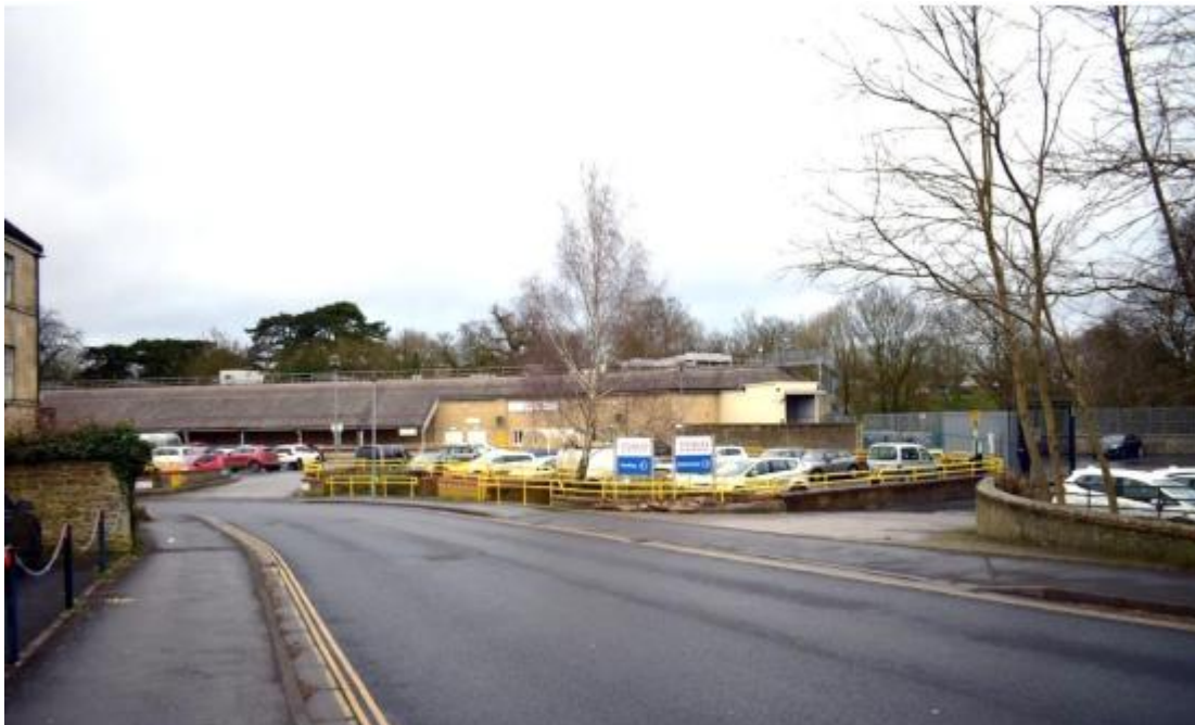
Figure 24: Image from Emery Lane looking to the application site and the former Tesco building, service yard and car park.
