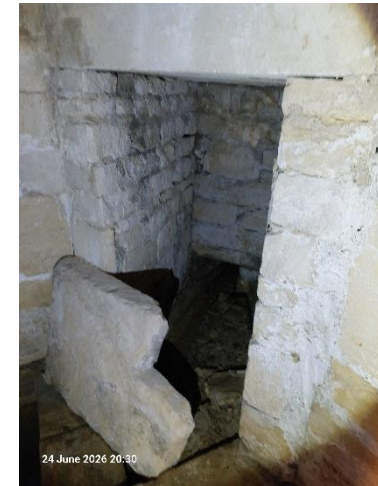
Photo 11: Well and stone features within the cellar
