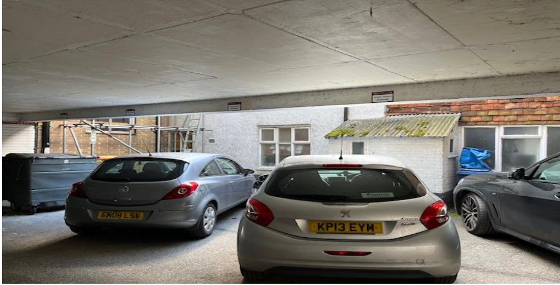
Photo 4: Undercroft parking and refuse bin storage
