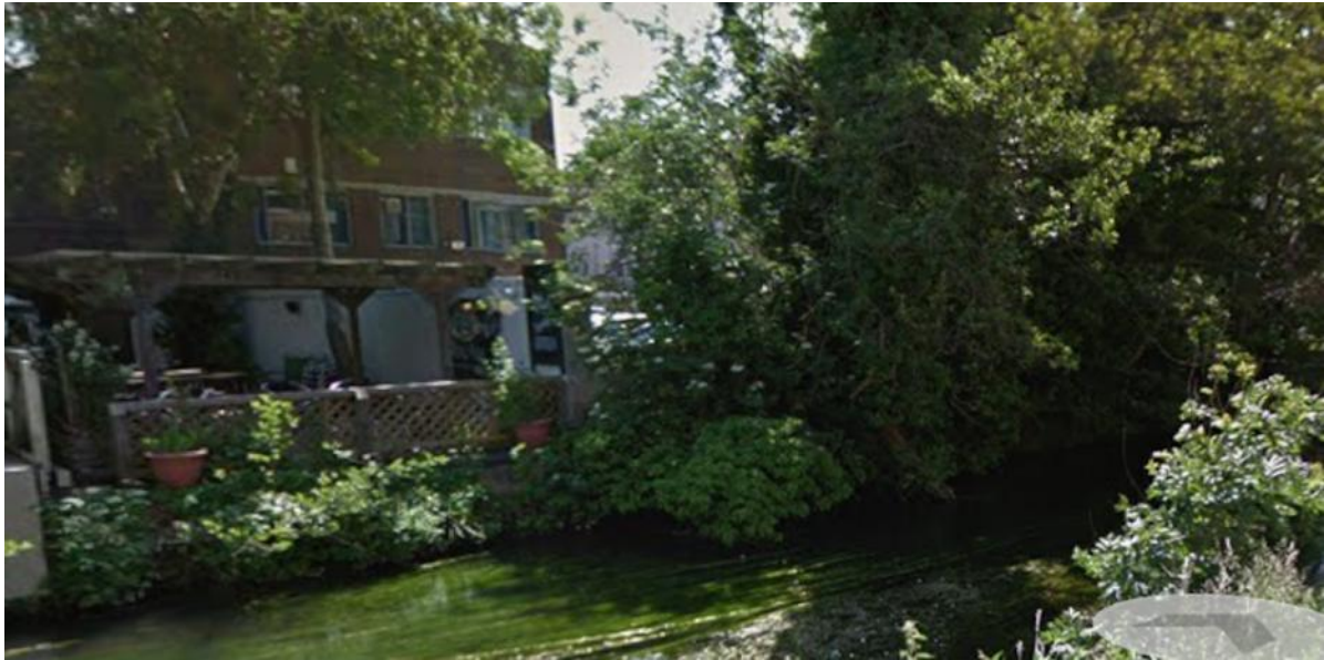
Photo 6: Subject property in background with pub garden in front backing onto river
