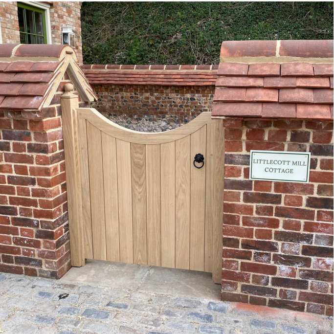
Image: Finished boundary wall for the mill cottage, used as the precedent for proposed mill house boundary wall.
