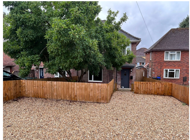
AS CONSTRUCTED - wide view from the hardstanding showing the transverse fencing, pedestrian opening and retained magnolia.
