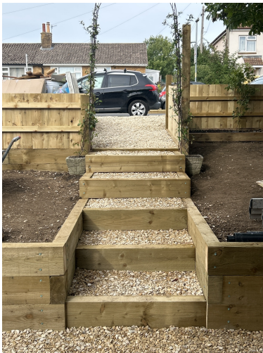
AS CONSTRUCTED - central stone steps/path and the pedestrian opening through the transverse timber fence.
