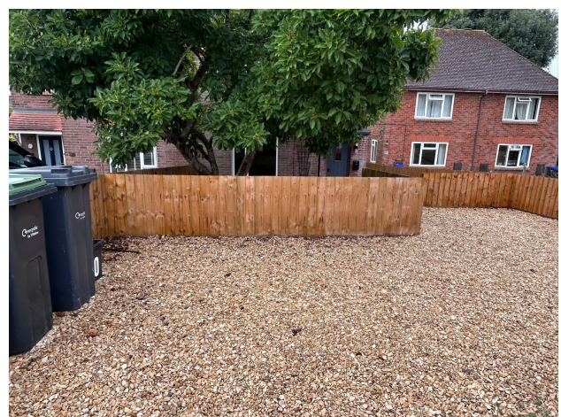
AS CONSTRUCTED - additional view of the permeable Cotswold buff stone hardstanding and timber fencing.
