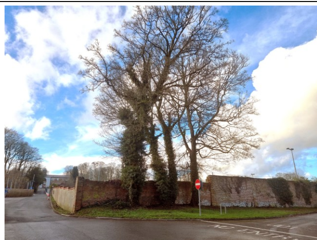
Photograph 16: Roadside view looking west.
