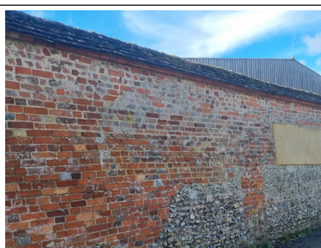
Photograph 14: Wall Section H with pitched wall coping.
