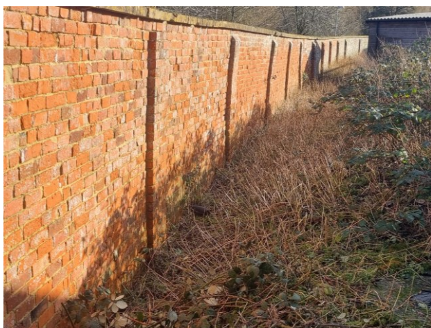
Photograph 7: Parcel 8 along the inside of the eastern wall.
