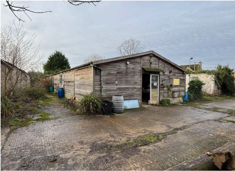
View of existing timber clad building
