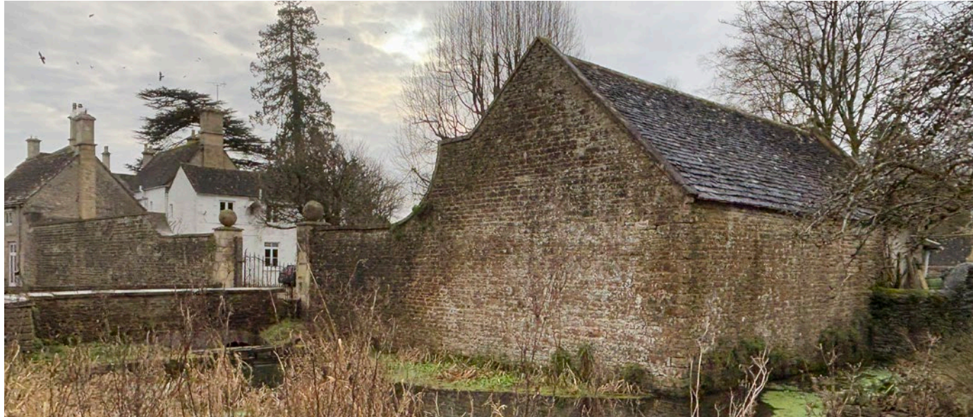
Barn forms ancillary to main house with gable facing street
