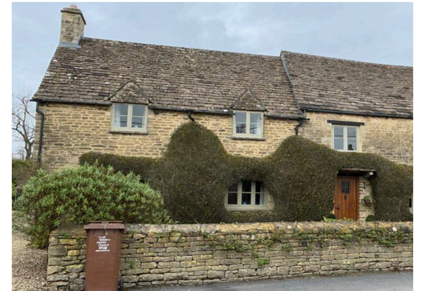
Row of cottages with dormers
