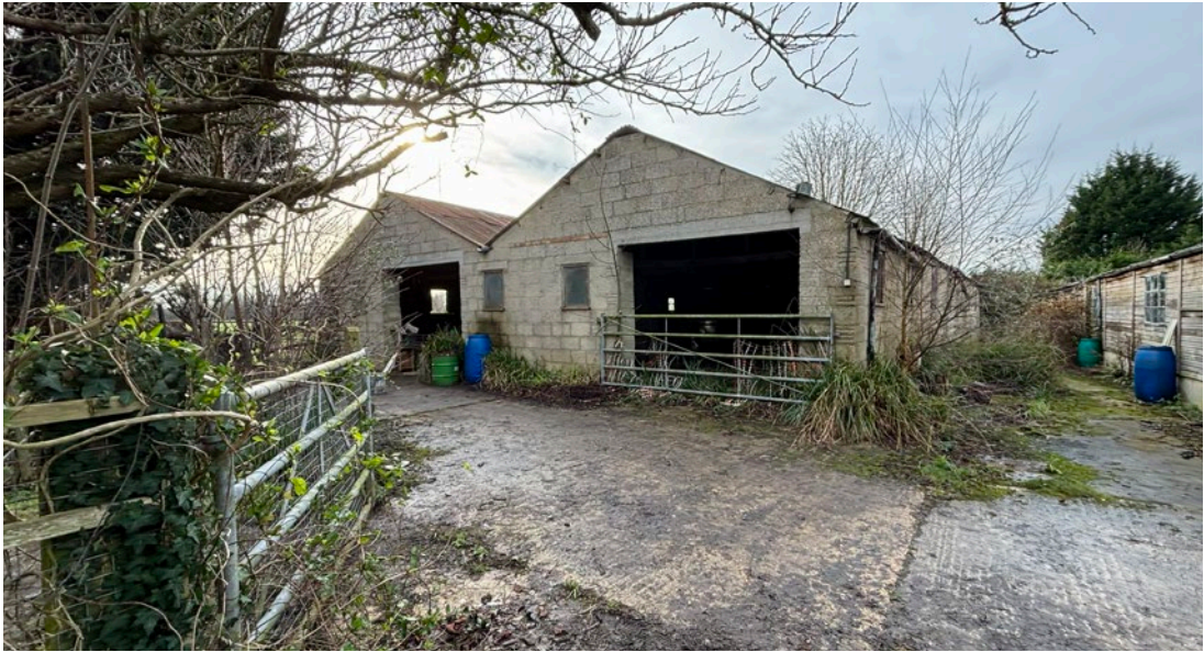
View of existing concrete block buildings
