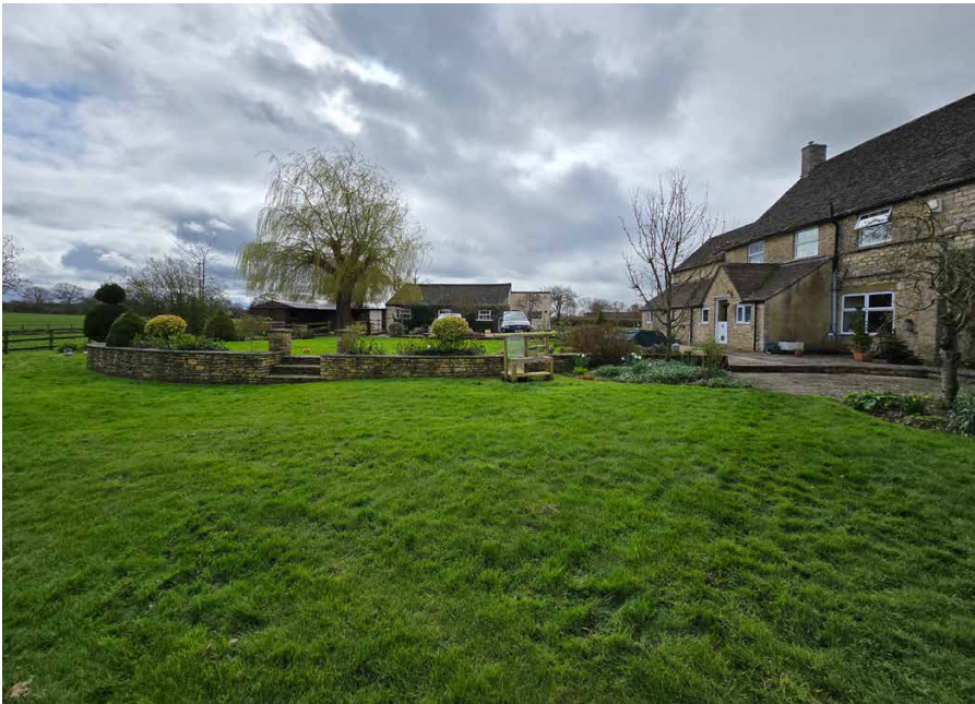
Rear main house elevation and outbuilding side elevation looking south from the garden
