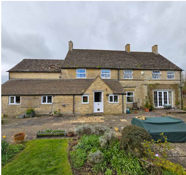
View of the East Elevation
