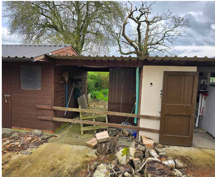
View of the timber stable block where it connects to the concrete barn/garage/workshop looking south
