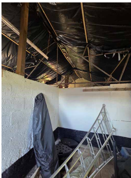
Internal view of the concrete block outbuilding
