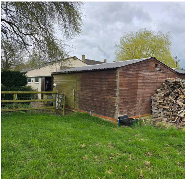
View of the timber stable block looking north west
