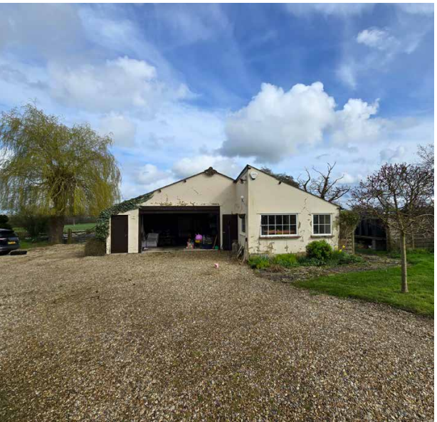
View of the West Elevation (Garage & workshop Side) looking south east
