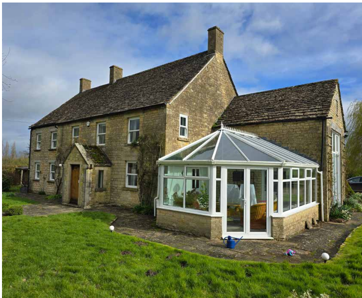
View of the West Elevation looking north east
