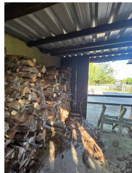
Internal view of the single lean-to which connects the timber stable block to the concrete block barn/garage/workshop
