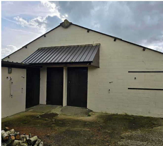
View of the concrete block outbuilding looking south west
