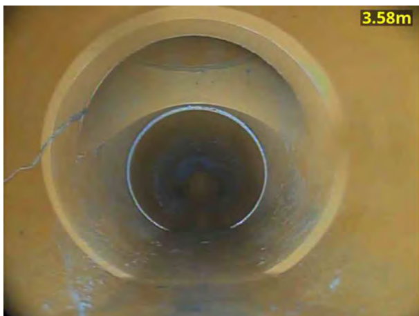
5, 00:00:59, 3.58 m Junction at 12 o'clock, 100mm dia
