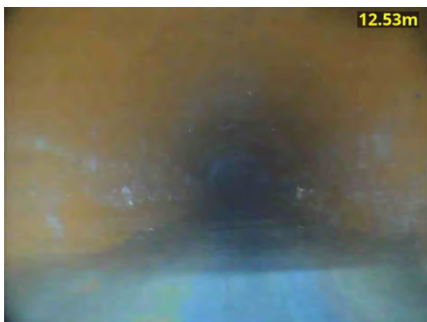
3, 00:01:25, 12.53 m Water level, 40% of the vertical dimension
