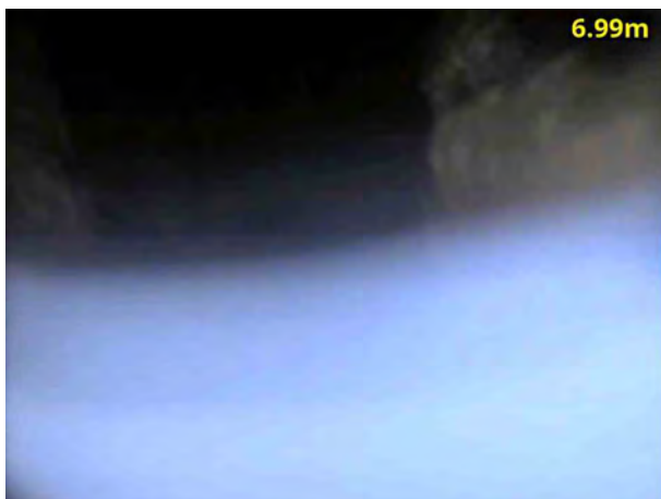
5, 00:01:22, 6.99 m Finish node, manhole, reference: MH12
