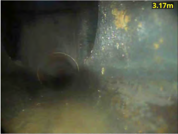
4, 00:00:38, 3.17 m Finish node, manhole, reference: MH16
