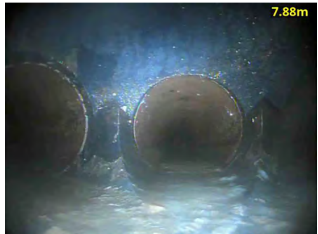
4, 00:01:09, 7.88 m Finish node, manhole, reference: MH11
