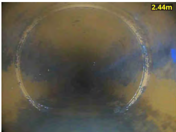
3, 00:00:28, 2.44 m Water level, 5% of the vertical dimension
