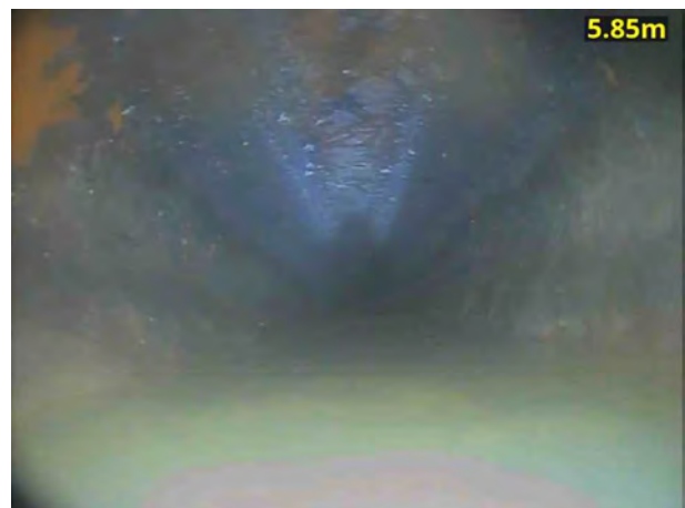
6, 00:00:57, 5.85 m Water level, 15% of the vertical dimension
