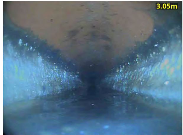
2, 00:01:10, 3.05 m Water level, 15% of the vertical dimension
