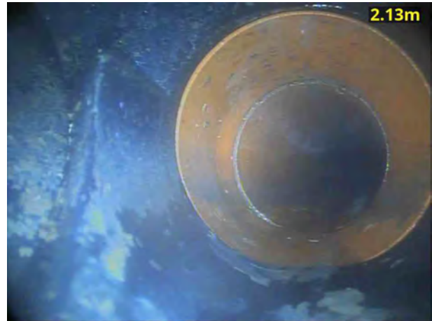
2, 00:00:35, 2.13 m Finish node, manhole, reference: MH14A
