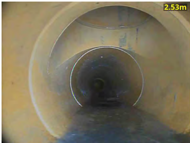
3, 00:00:52, 2.53 m Junction at 12 o'clock, 100mm dia
