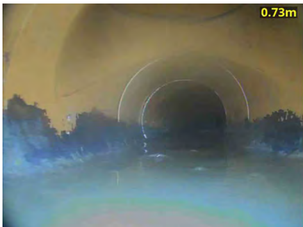
3, 00:00:30, 0.73 m Junction at 12 o'clock, 100mm dia
