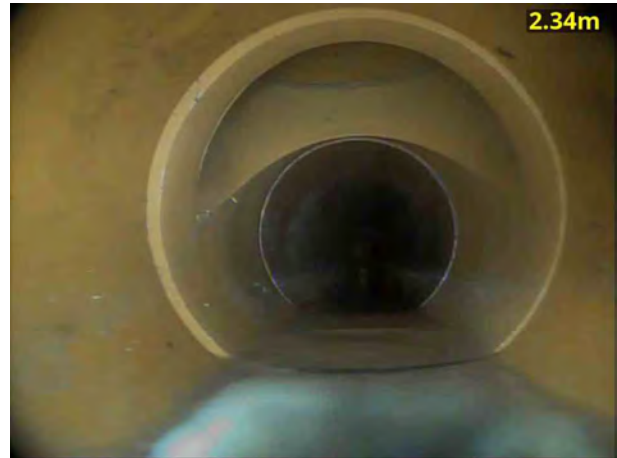
2, 00:00:27, 2.34 m Junction at 12 o'clock, 100mm dia
