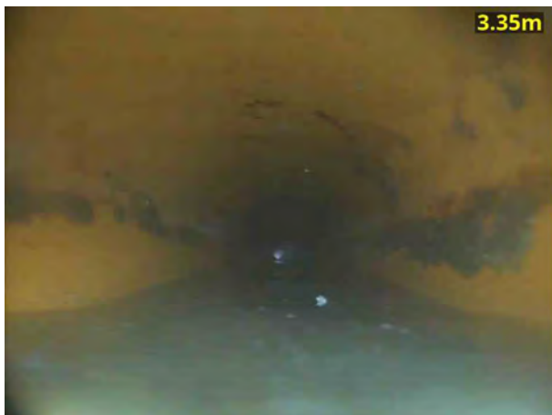
3, 00:00:36, 3.35 m Water level, 20% of the vertical dimension
