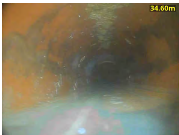
5, 00:03:57, 34.60 m Water level, 50% of the vertical dimension
