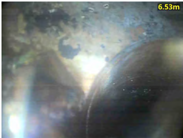
3, 00:01:08, 6.53 m Finish node, manhole, reference: MH7
