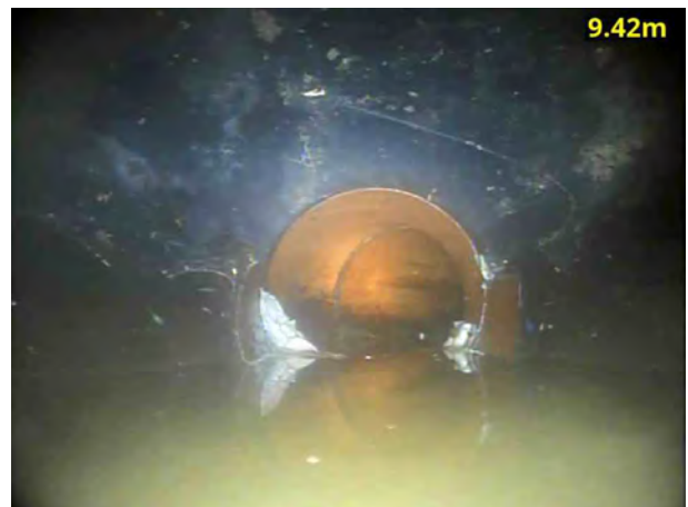
4, 00:01:26, 9.42 m Finish node, manhole, reference: MH6
