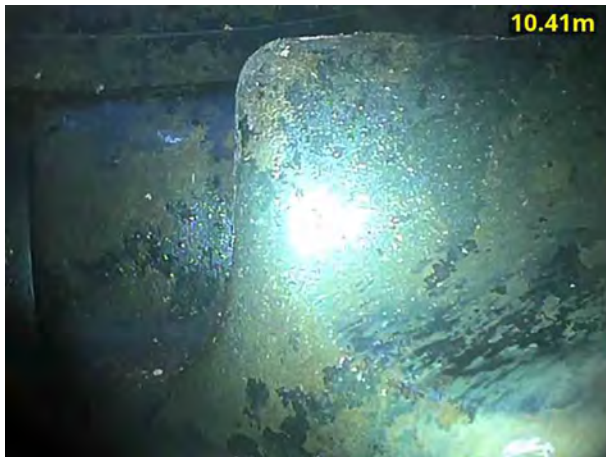
5, 00:01:28, 10.41 m Finish node, manhole, reference: MH3
