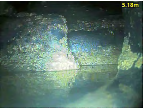
3, 00:00:43, 5.18 m Finish node, manhole, reference: MH12
