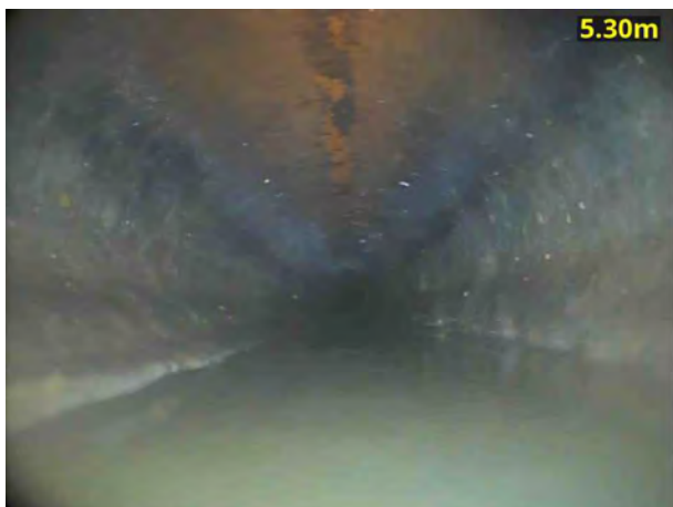
5, 00:00:53, 5.30 m Water level, 10% of the vertical dimension
