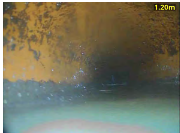
4, 00:00:37, 1.20 m Water level, 15% of the vertical dimension
