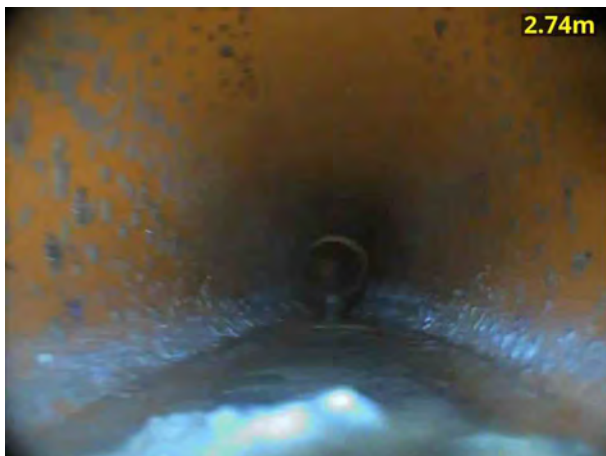
3, 00:00:31, 2.74 m Water level, 10% of the vertical dimension
