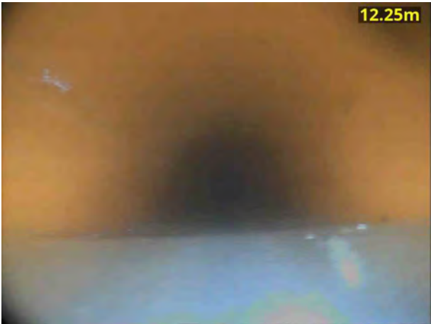
9, 00:01:54, 12.25 m Water level, 20% of the vertical dimension
