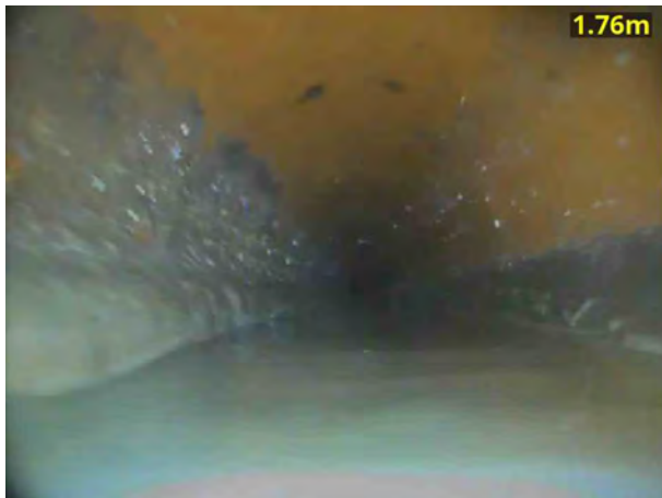
3, 00:00:27, 1.76 m Water level, 20% of the vertical dimension
