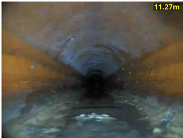
3, 00:01:29, 11.27 m Water level, 5% of the vertical dimension
