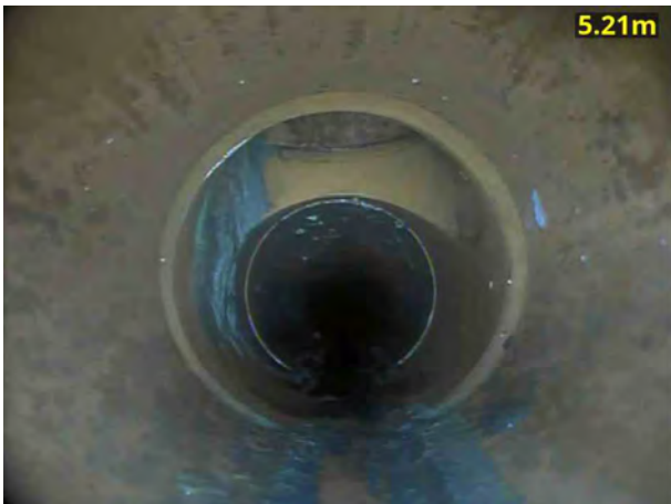
3, 00:00:48, 5.21 m Junction at 12 o'clock, 100mm dia
