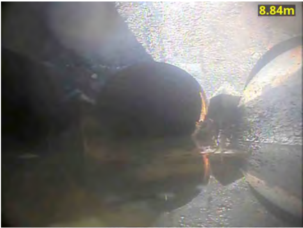
8, 00:01:37, 8.84 m Finish node, manhole, reference: MH5
