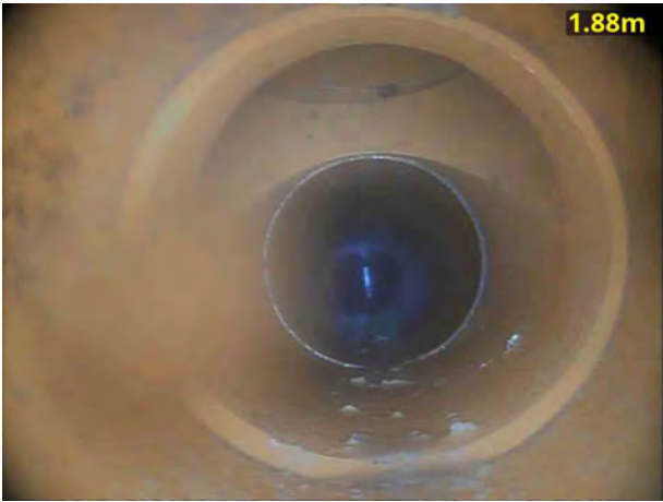
2, 00:00:22, 1.88 m Junction at 12 o'clock, 100mm dia
