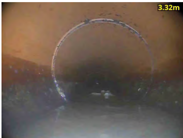
3, 00:00:30, 3.32 m Water level, 15% of the vertical dimension
