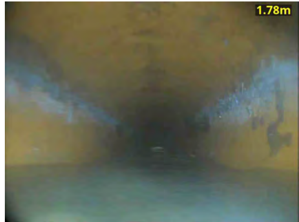
2, 00:00:24, 1.78 m Water level, 15% of the vertical dimension
