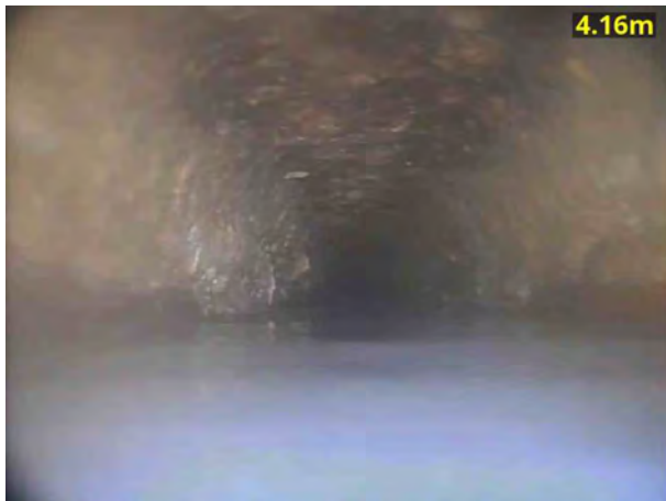
3, 00:00:40, 4.16 m Water level, 30% of the vertical dimension
