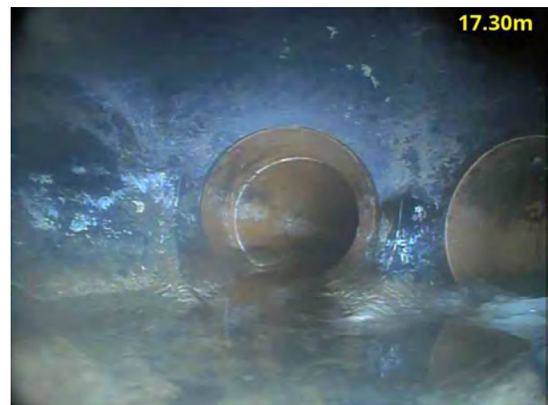
6, 00:02:20, 17.30 m Finish node, manhole, reference: MH8
