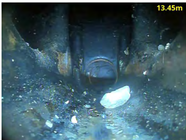
5, 00:01:46, 13.45 m Finish node, manhole, reference: MH14
