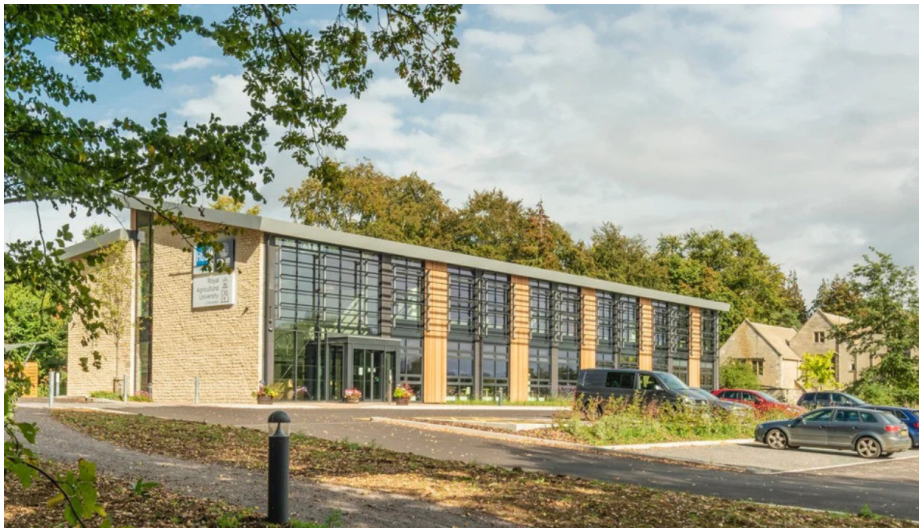
4. The Alliston Centre- Glazing & Entrance Precedent
