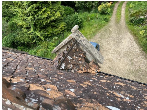
Figures 18, 19 and 20 – The roof is generally in a very poor condition with no roofing felt, poor levels of insulation, numerous slipped or missing tiles and defects to stonework, leadwork etc.
