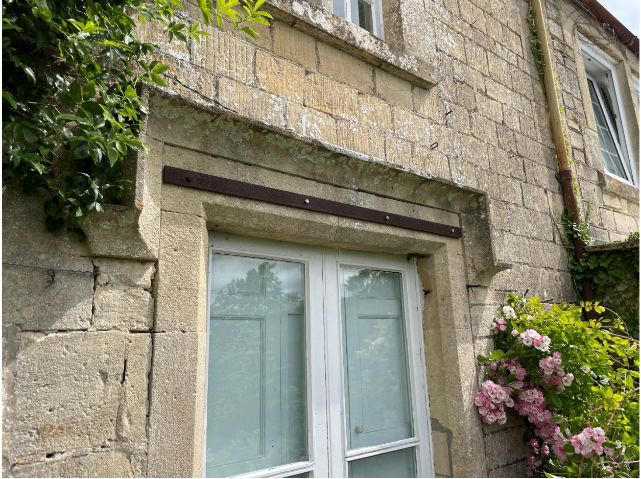
Figure 17 - A metal strap has been added as a structural repair to the lintel on the south elevation.
