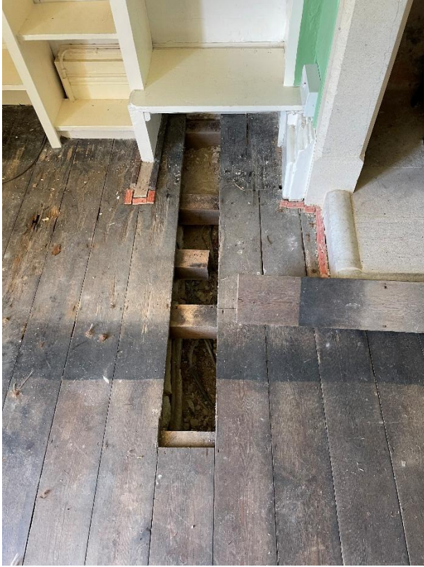
Figures 27 and 28 – pine floorboards have been lifted to show floor construction. Some fire places such as Room 3 (proposed kitchen) have been previously altered.
