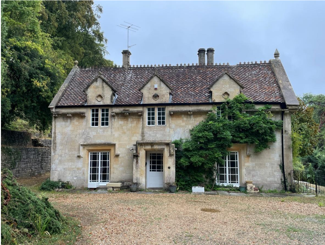
Figure 41 – The west elevation.
