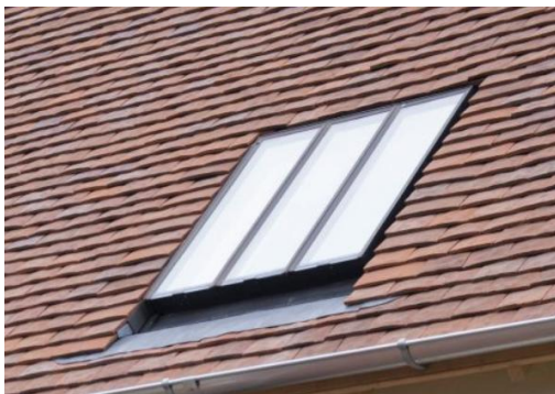
Figures 33, 34, 35 and 36 – Steico wood fibre insulation, Victorian ogee cast aluminum gutters, handmade natural clay club tiles in dark antique and conservation roof lights.
