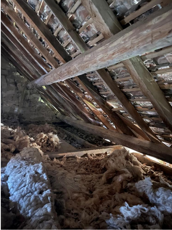
Figures 18, 19 and 20 – The roof is generally in a very poor condition with no roofing felt, poor levels of insulation, numerous slipped or missing tiles and defects to stonework, leadwork etc.
