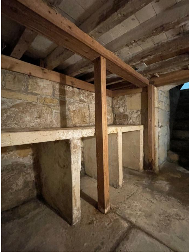
Figures 29 and 30 – The original stone throwls and spring to the cellar, which still provides the house with drinking water as it is not connected to the main supply.
