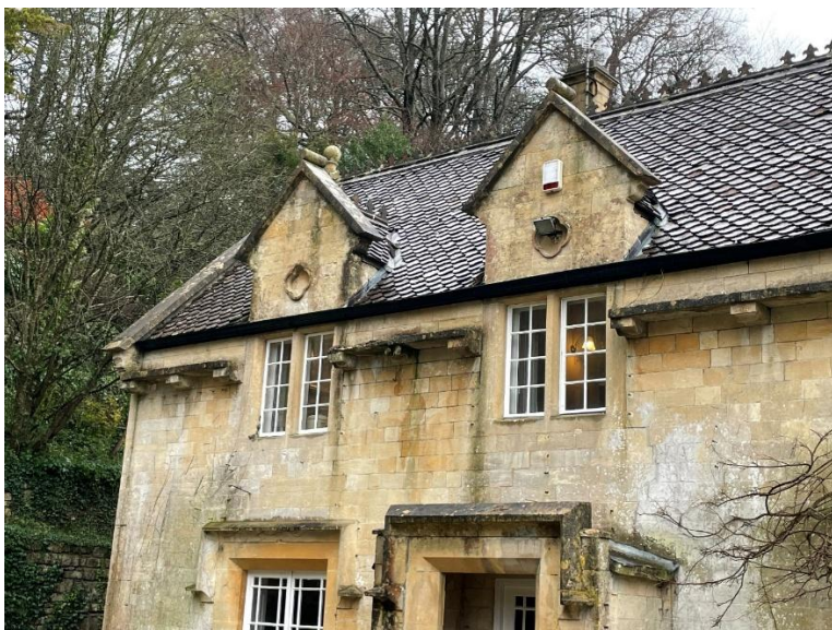
Figures 13, 14, 15 and 16 – Examples of deterioration of stonework to south, north and west elevations. An historic doorway to the west elevation was infilled as part of the 19 th century improvements and there appears to be a blocked up window to the north elevation.
