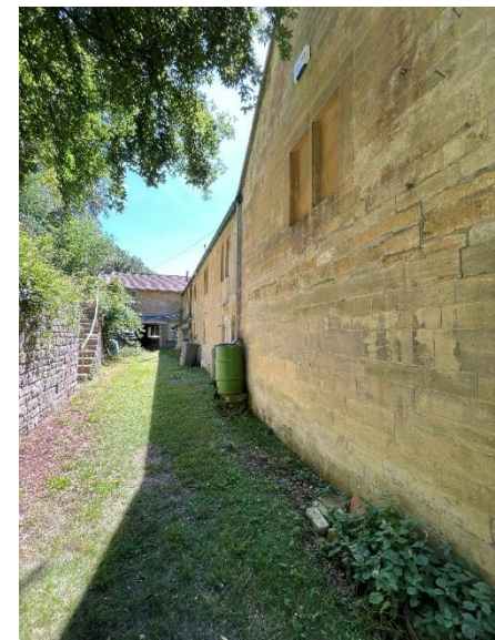
Figures 13, 14, 15 and 16 – Examples of deterioration of stonework to south, north and west elevations. An historic doorway to the west elevation was infilled as part of the 19 th century improvements and there appears to be a blocked up window to the north elevation.
