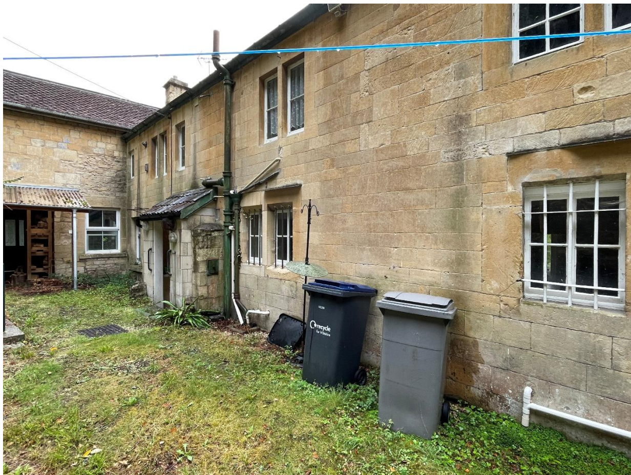
Figure 43 – The north elevation can be clearly read as the less important in terms of aesthetic value.
