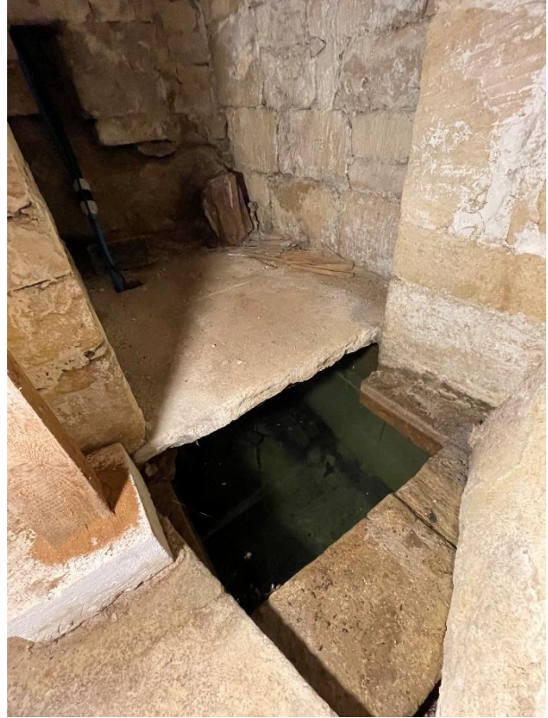
Figures 29 and 30 – The original stone throwls and spring to the cellar, which still provides the house with drinking water as it is not connected to the main supply.
