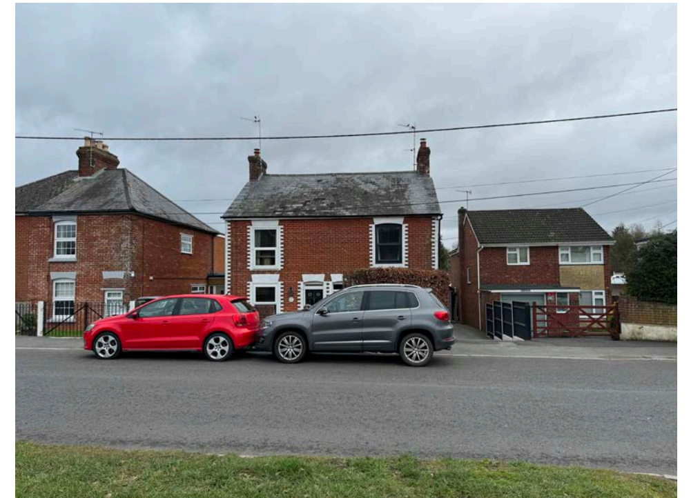
Pair of semi-detached houses in red brick with quions and windows expressed with painted brick detail. Detached modern red brick house with stone detail panel to right, set further back from the road, breaking from the symmetrical elevations of adjacent houses
