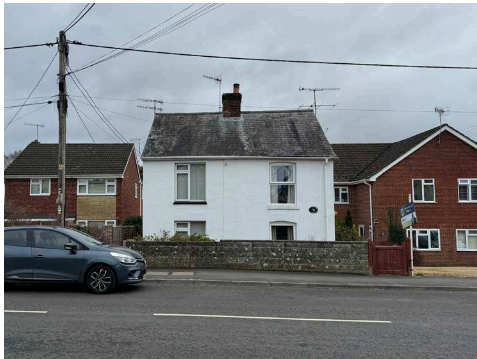
Pair of painted render semi-detached houses with slate roof and simple windows
