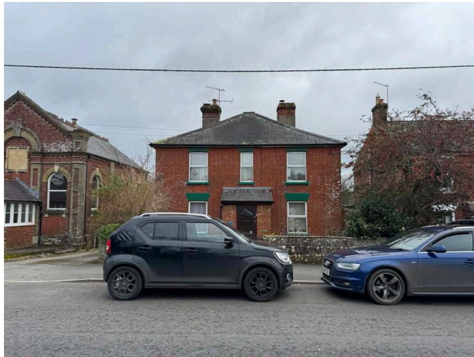
Symmetrical detached dwelling of red brick and slate roof. Flat brick arches over windows.
