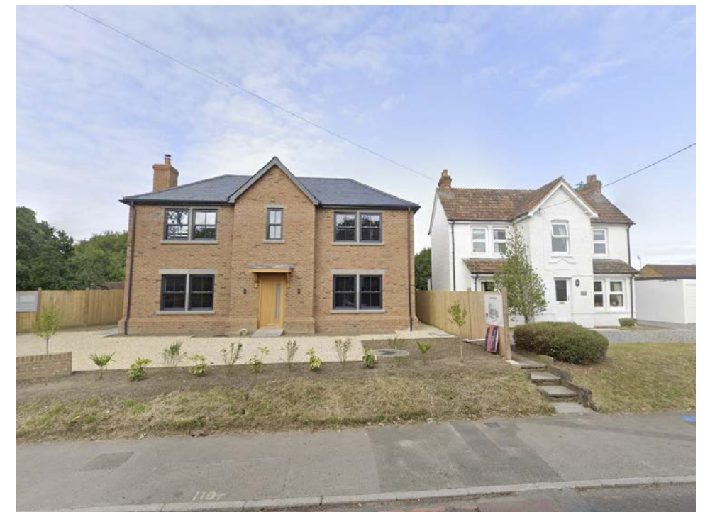
Recently completed new build dwelling with brown brick and slate roof. Follows the typology of balanced and symmetrical elevational treatment
