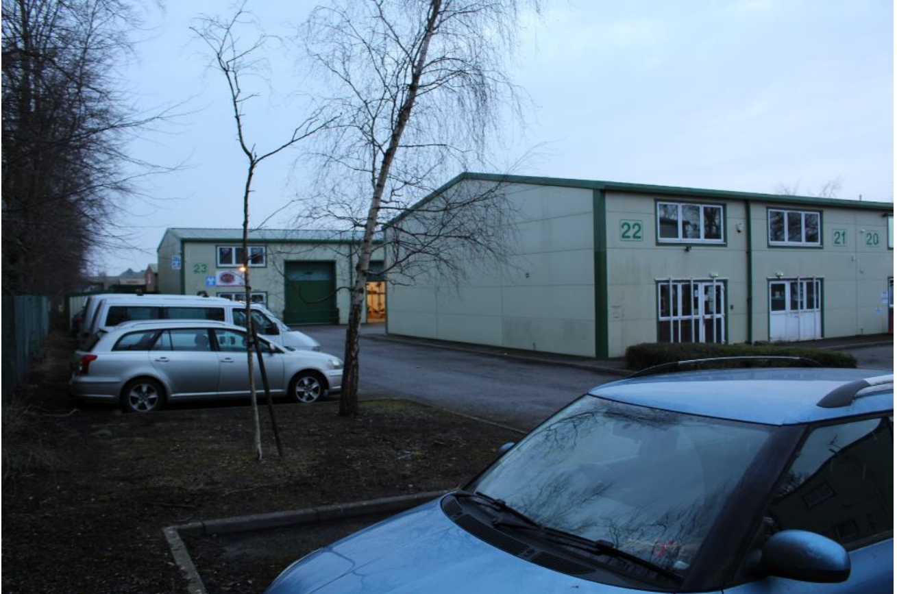
Photograph 10: View west toward the proposed development area from the northern boundary of the airfield Conservation Area, with the listed workshops (1391602) behind, showing modern development disrupting intervisibility.
