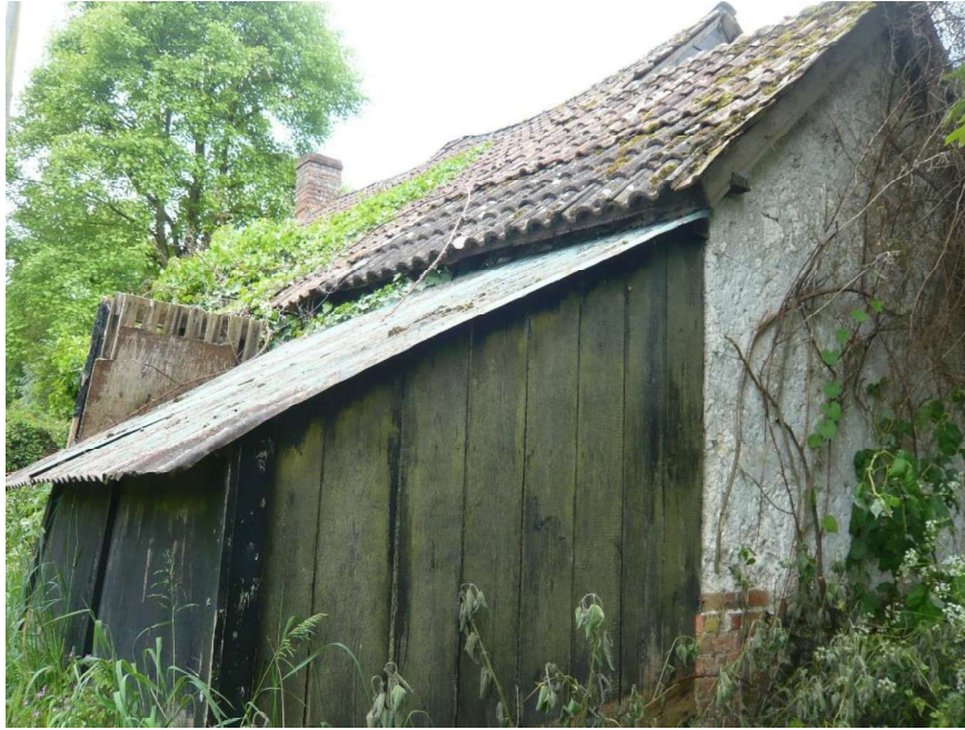
Fig.6 Lean-to on the rear of the building
