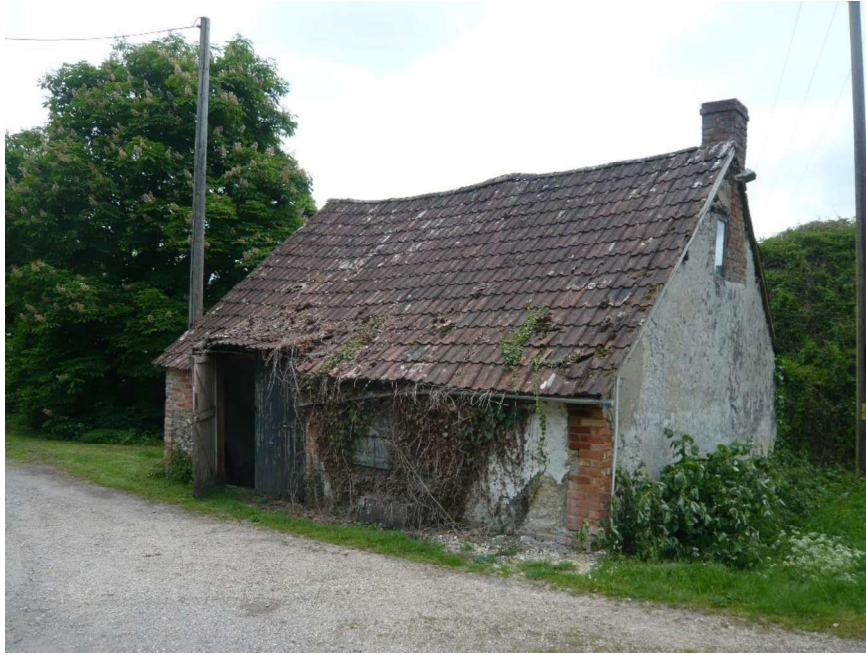
Fig.4 View from the south
