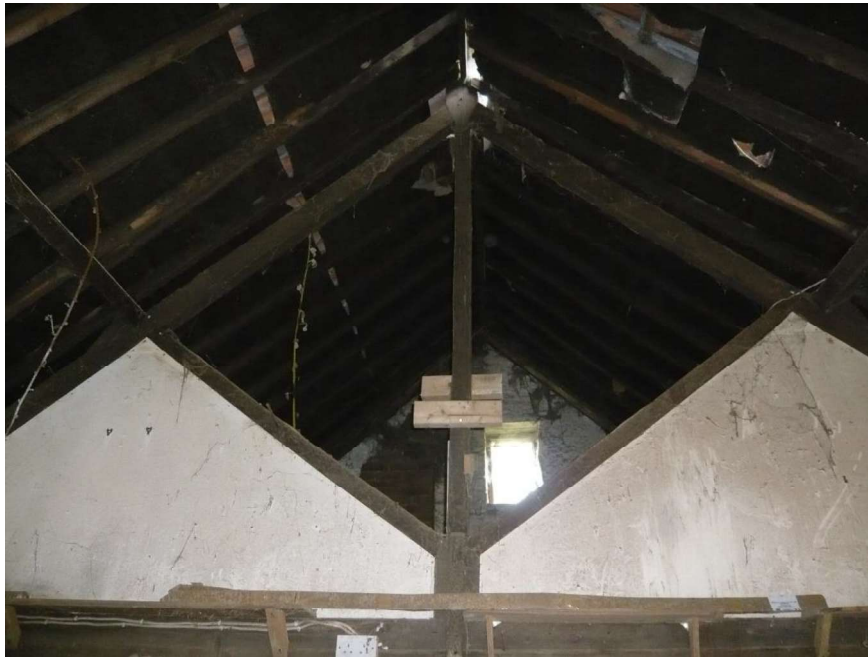
Fig.9 King-post truss with plaster infill below the struts
