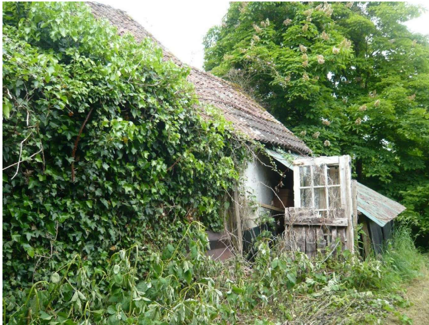
Fig.7 View along the back of the building
