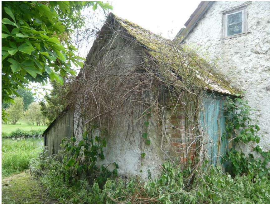
Fig.5 Shed structure on the northern end of the building
