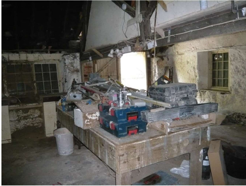
Fig.8 Interior of the building – concrete floor, cob walls and king-post truss
