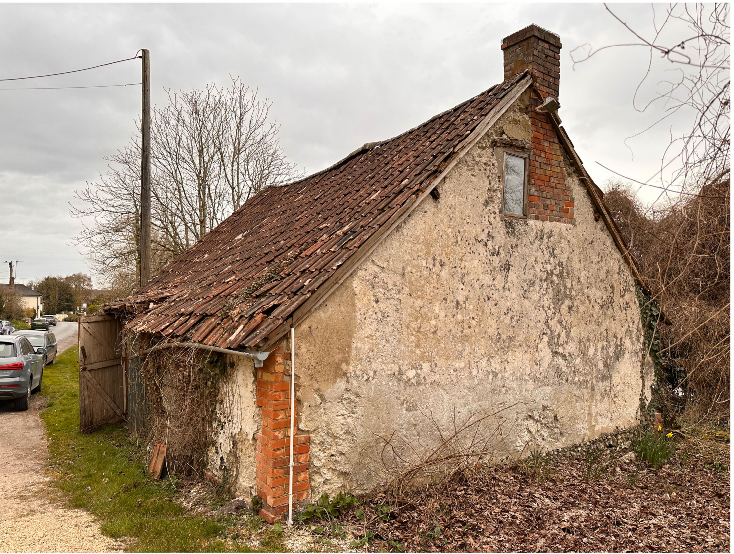
View of south elevation
