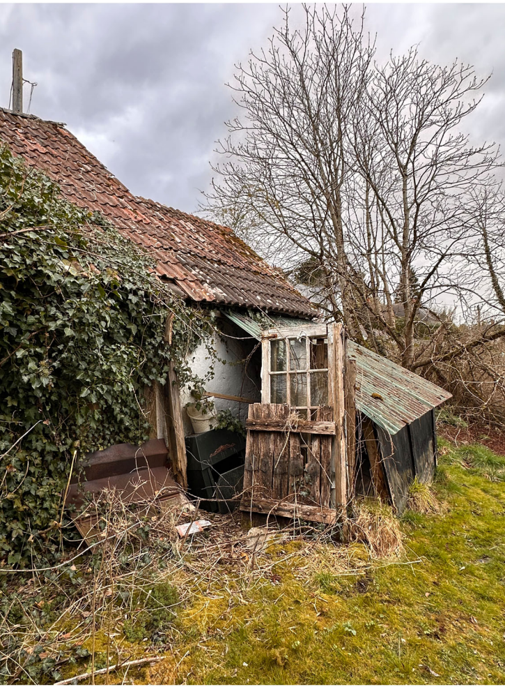
View of lean to and ivy covered east wall
