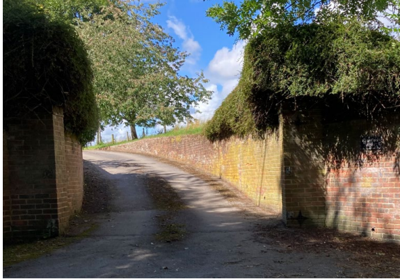
Curved walls at entrance to No. 69
