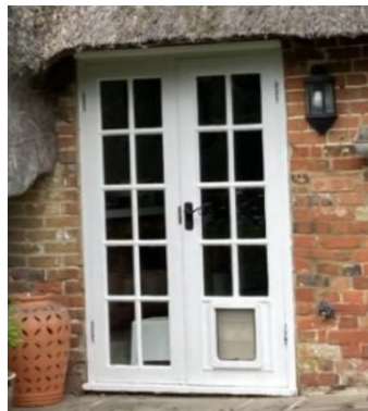
63 Hawthorn Cottage Patio Doors
