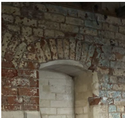
Existing Internal Recess & Archway
