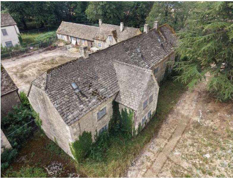
Plot 53– Imitation Cotswold concrete slates on outer roof slope
