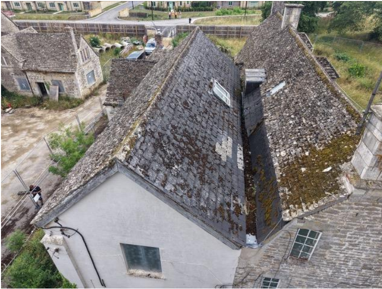
Plot 55 (Farmhouse) – Artificial Welsh slates on inner roof slope. Existing verge detail can be maintained using artificial Welsh slates on both slopes of 19 th century wing.
