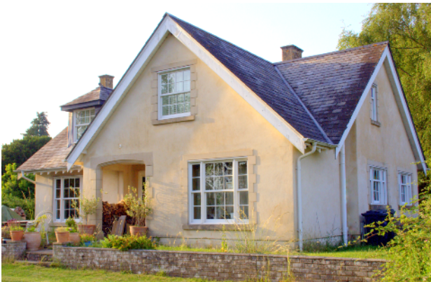
Figure 1. Brandicove – a chalet-bungalow style house of rendered elevations and cast stone features under a natural slate roof
