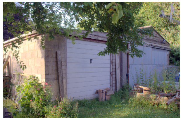
Figure 2. Existing Garages – concrete block elevations under a corrugated sheet roof
