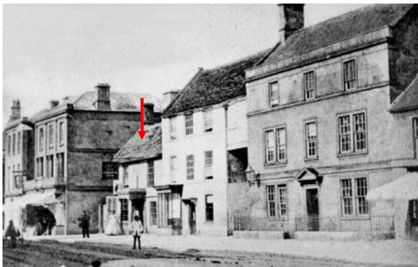
Figure 1 Late 19 th century photograph of High Street, Melksham showing at modest two storey thatched house on the site of No 12.
