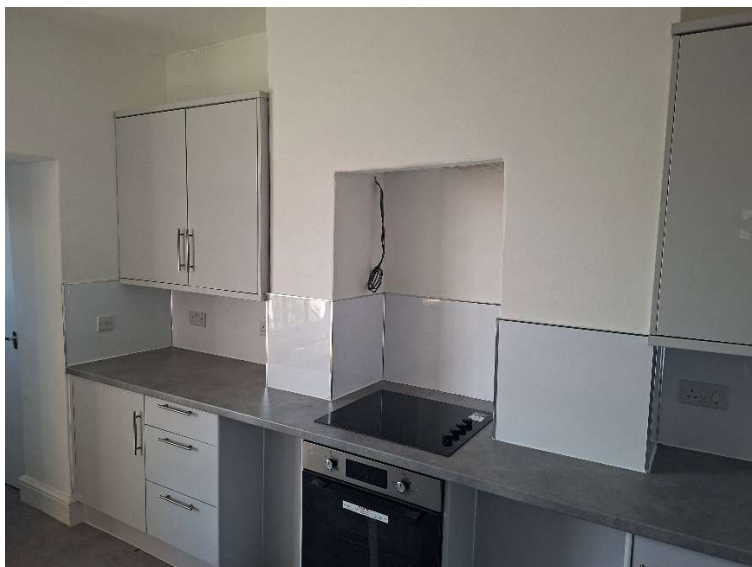
Figure 4 The kitchen at first floor level with the enlarged fireplace opening.
