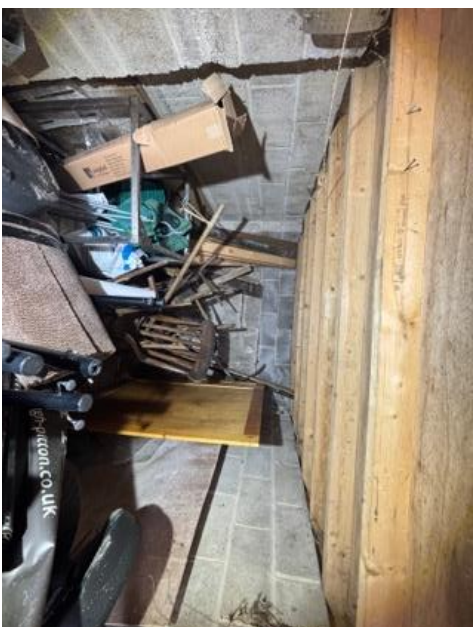
Internal space of garage
