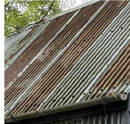
Corrugated tin roof
