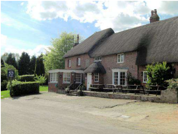
View facing pub from south east of Gores Lane
