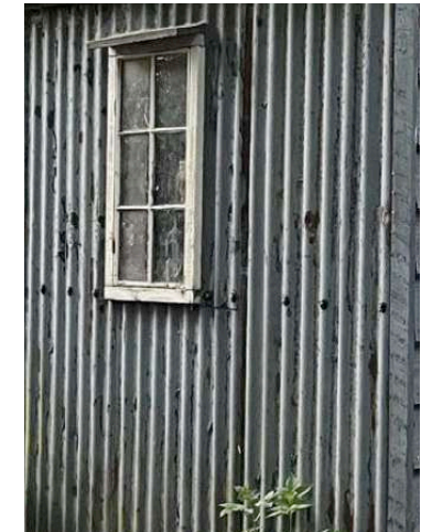
Corrugated tin cladding
