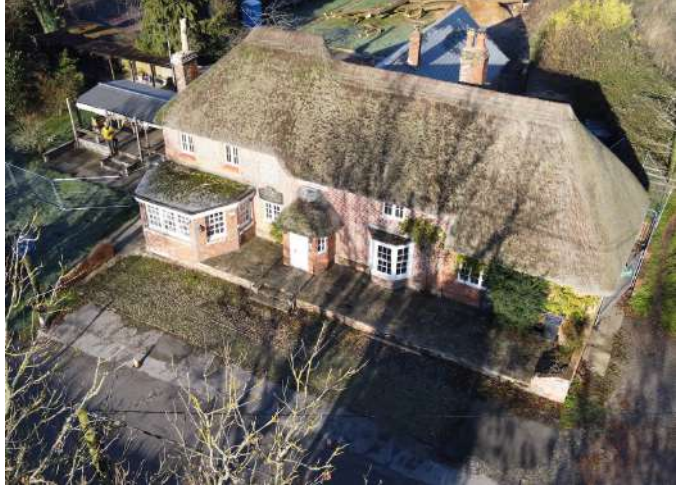
Arial view of pub from the south east
