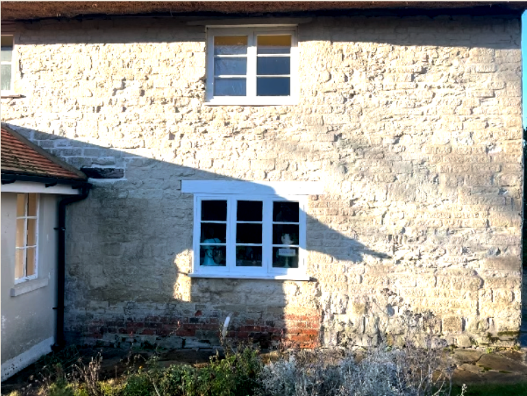
Figure 7 – South elevation, brickwork repair to base of stone wall. Historic front door lintel remains behind C20 porch extension
