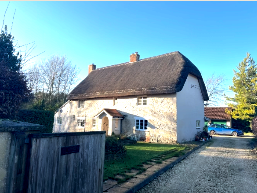
Figure 2 – Entrance onto site, South elevation with 1973 porch and C20 extension to the west gable
