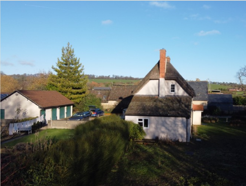
Figure 3 – West elevation of Quemerford Gate Cottage, C20 extension containing office and bathroom
