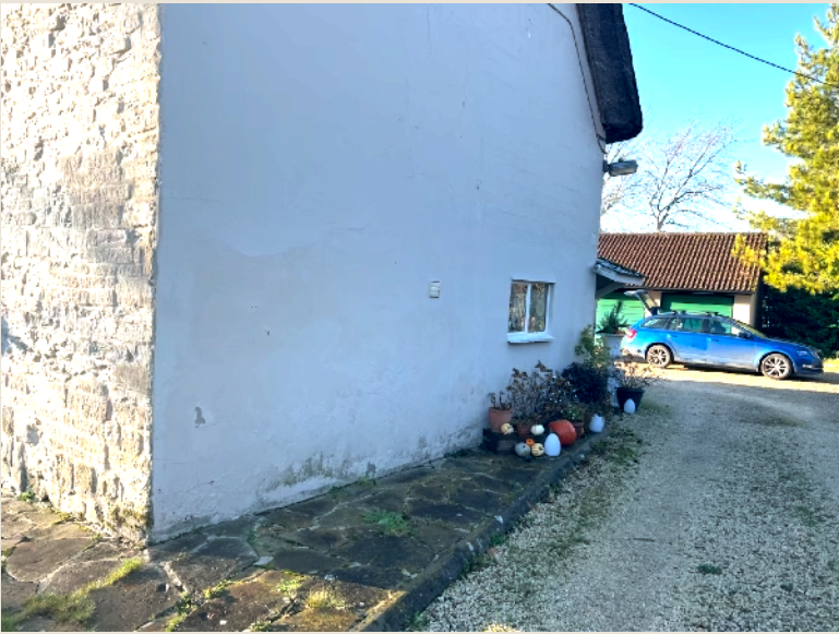
Figure 8 – East elevation, with modern concrete block resurfacing repairs to chalk stone
