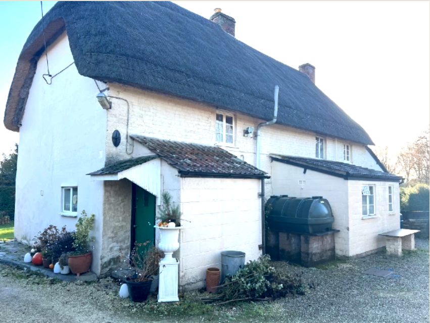
Figure 1 – North-east view of Quemerford Gate Cottage, two C20 extensions
