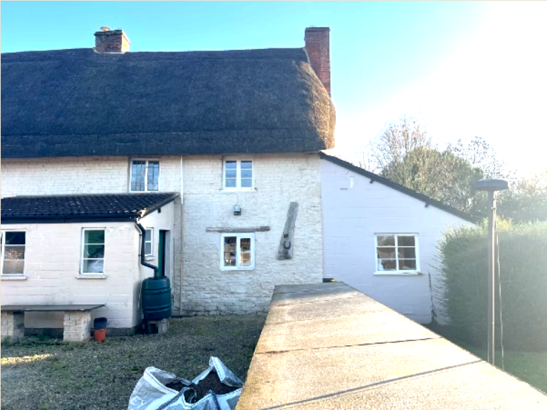
Figure 6 – North elevation, modern facings repair to brickwork.
