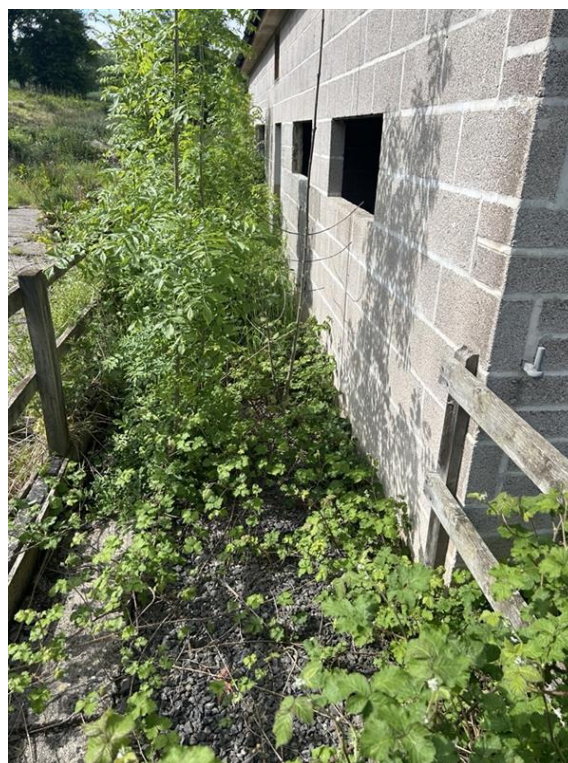
Figure 3-8 Western Barn Perimeter French Drain
