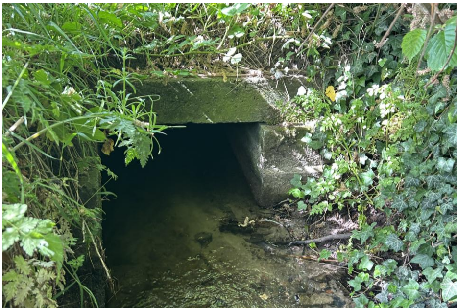
Figure 3-1 Brick Culvert Upstream Inlet
