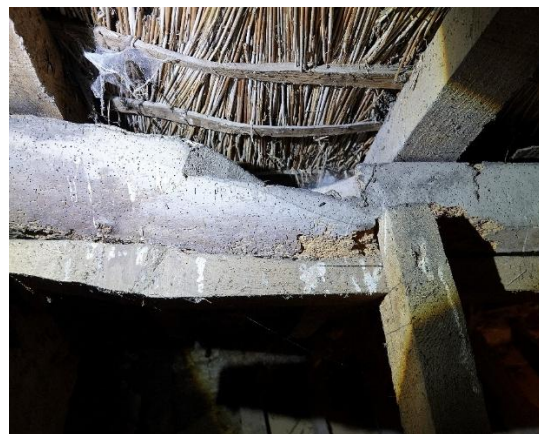
Figs.92 & 93 – vacant housings for a lost windbrace on the purlins near the NE end wall (left) the NW purlin; (right) the SE purlin
