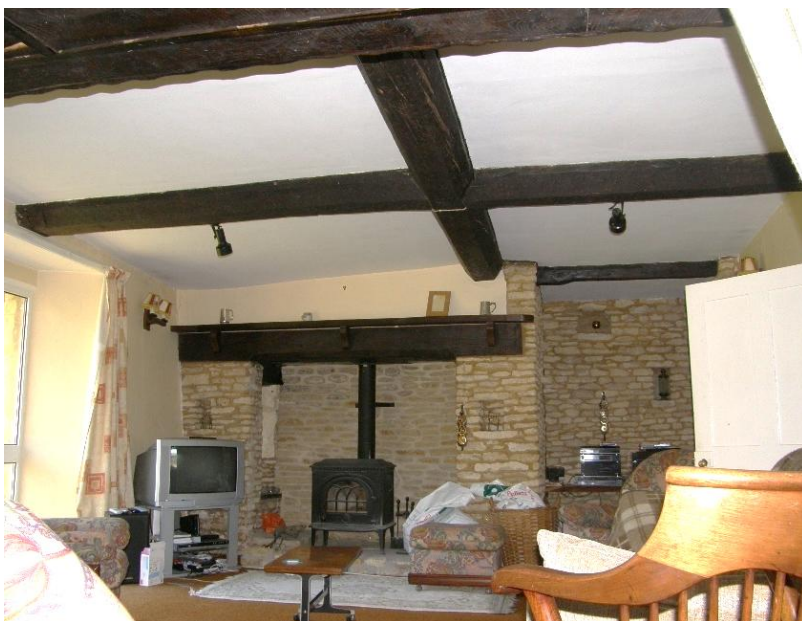
Fig.22 Little Lype Farmhouse, Charlton, near Malmesbury, dating to the earlier 17 th century showing plain quartered ceiling and empty recess to right for former newel stair
