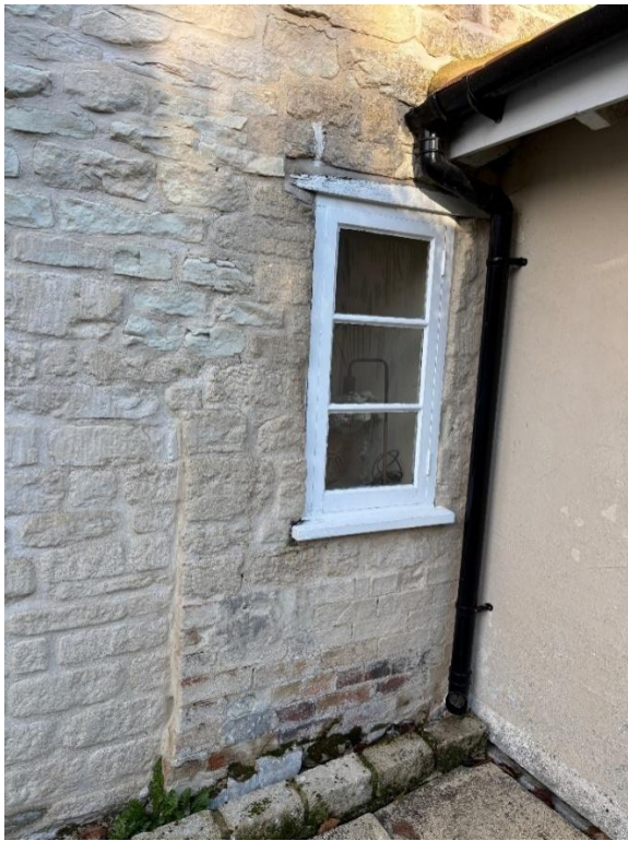
Fig.26 Detail of brickwork repair to wall to left of front porch
