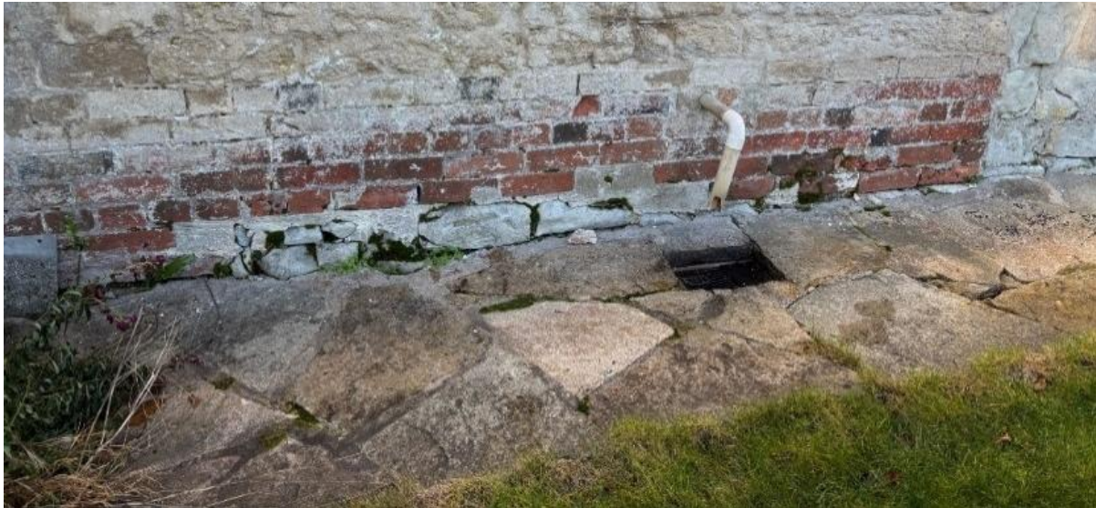
Fig.24 Brick repair of wall footing in late 19 th century or early 18 th century using a form of English garden wall bond coursing. Note queen closer at right-hand end to bring the brickwork to a common edge. Note 'crazy paving' in front surrounding drain.
