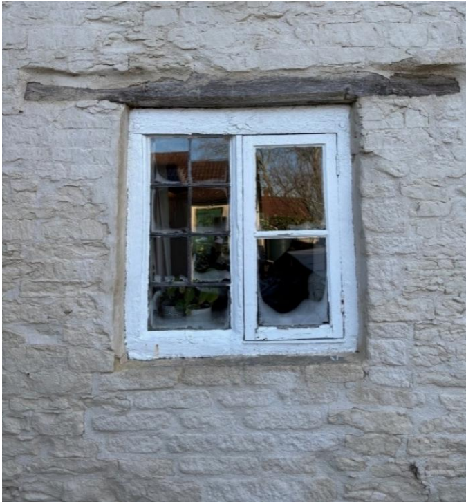
Fig.34a Ground floor window to west cottage with original pegged frame, chamfered and stopped lintel, and early leaded glazing. Patch of renewed stonework below window
