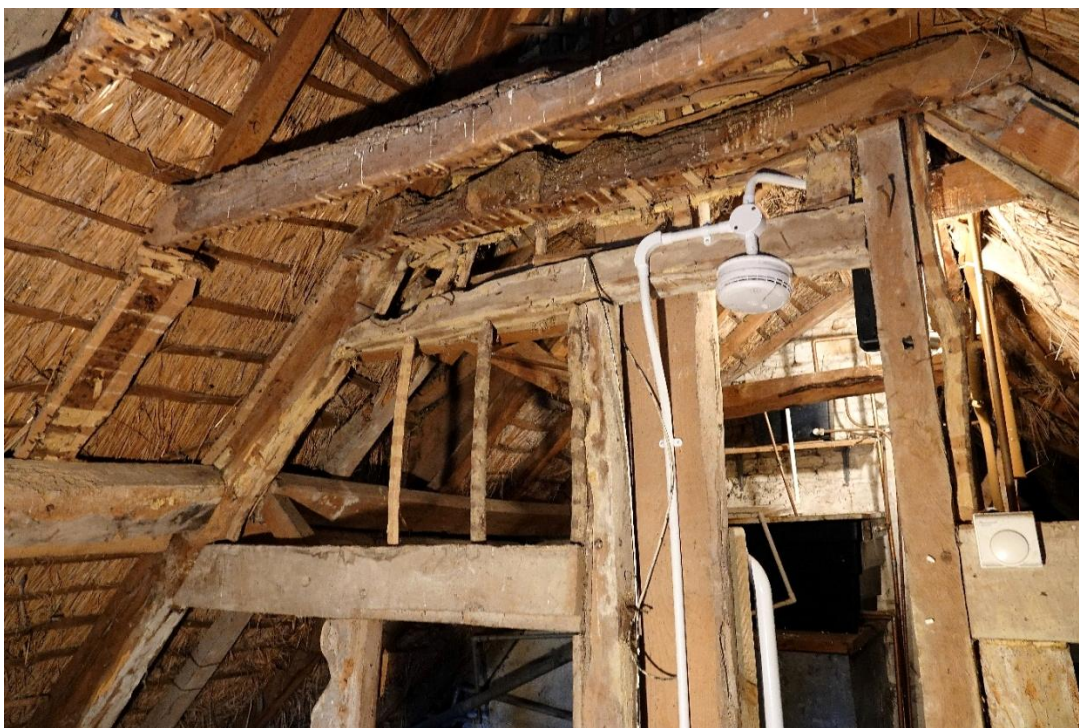
Fig.72 – A view of Truss T1 from the SW side
