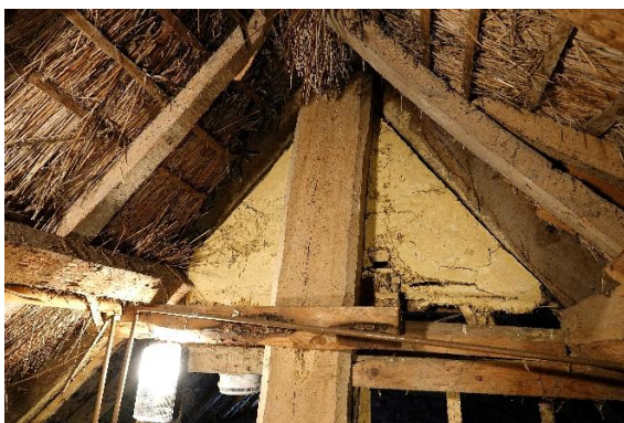
Figs. 75 & 76 – (left) plastered face of the upper part of T1, facing to the central stack; (right) the unplastered face to the end wall
