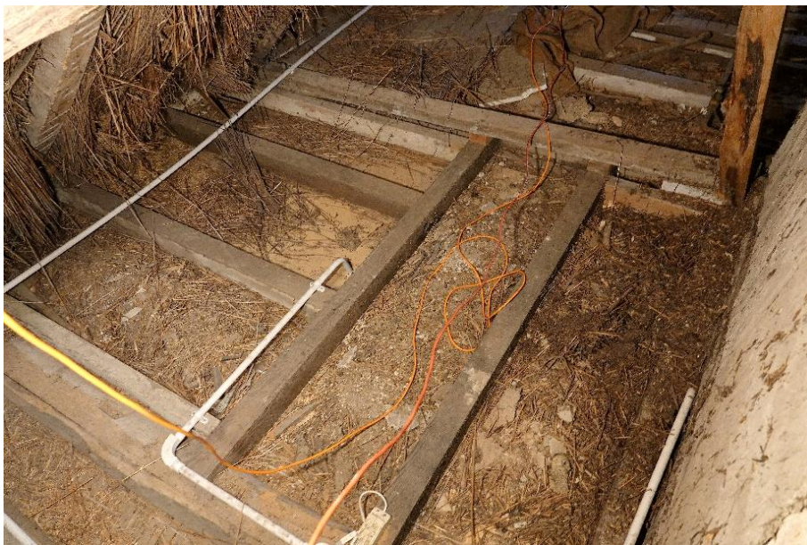
Fig.82 – the area in front of the central stack where the stairs ascended. Note the use of heavy floor joists to provide lateral restraint
