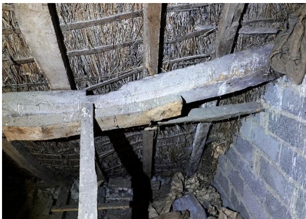
Figs.92 & 93 – vacant housings for a lost windbrace on the purlins near the NE end wall (left) the NW purlin; (right) the SE purlin
