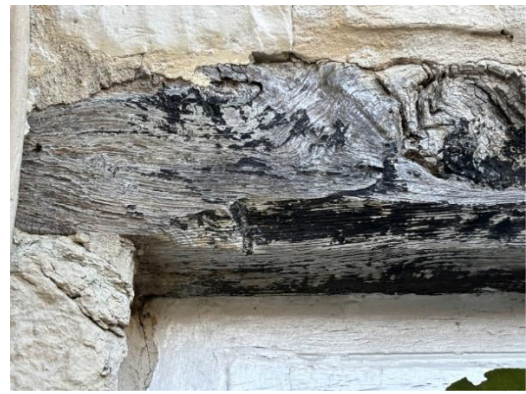
Fig.31 Rear window to east cottage with chamfered and stopped lintel
