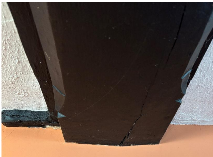
Fig.61 West end of axial beam in bedroom 1. Note accidental uneven spacing of stops
