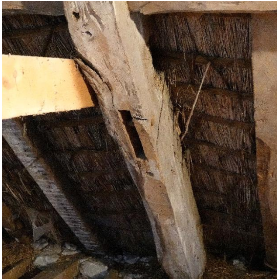
Figs.89 & 90 – details of T2; (left) vacant mortise for the missing collar; (right) the apex detail
