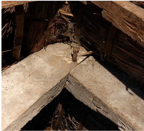
Figs.89 & 90 – details of T2; (left) vacant mortise for the missing collar; (right) the apex detail
