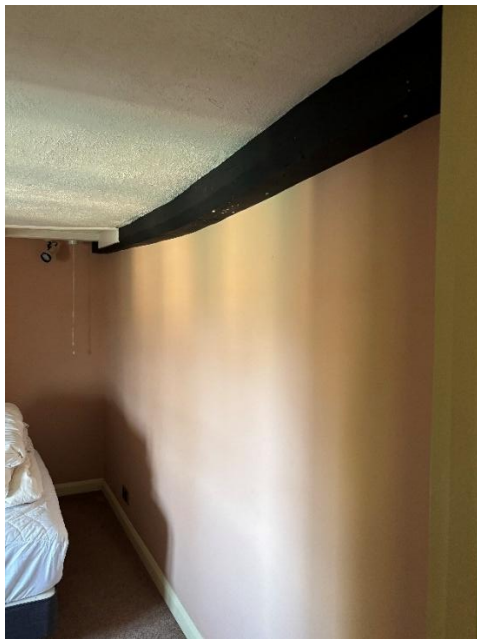
Fig.53 Chamfered axial beam between bedrooms 2 & 3, seen from bedroom 2
