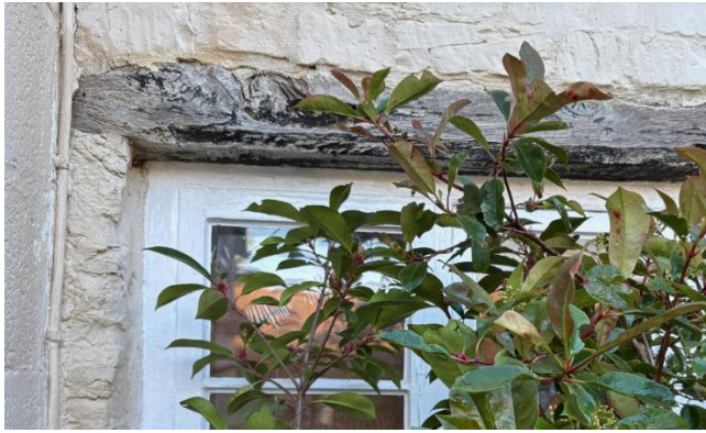
Fig.31 Rear window to east cottage with chamfered and stopped lintel
