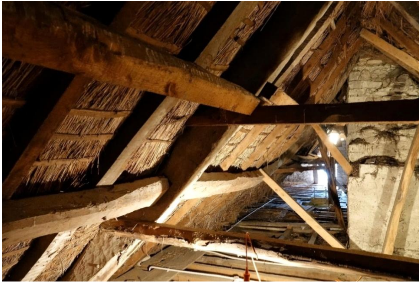
Fig.83 – a view from NE of the central stack along the front of the roof space looking SW to the far end wall. In the foreground is T2. Note the extensive propping necessary. The upper purlin and the collars visible are all later additions
