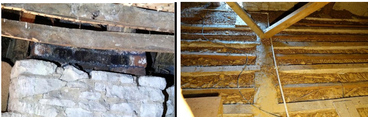
Figs.65 and 66 – (left) detail of the end gable stack showing brick courses (right) floor with spine beam in the end bay
