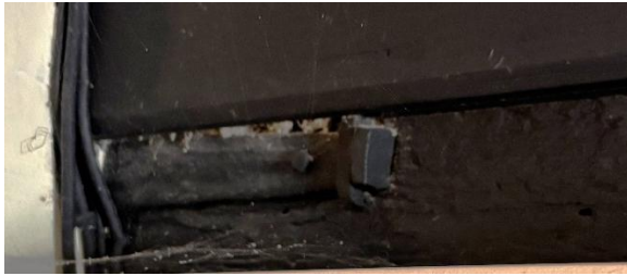
Figs.47 & 48 Straps for wall anchors at south and north ends of west gable end beam
