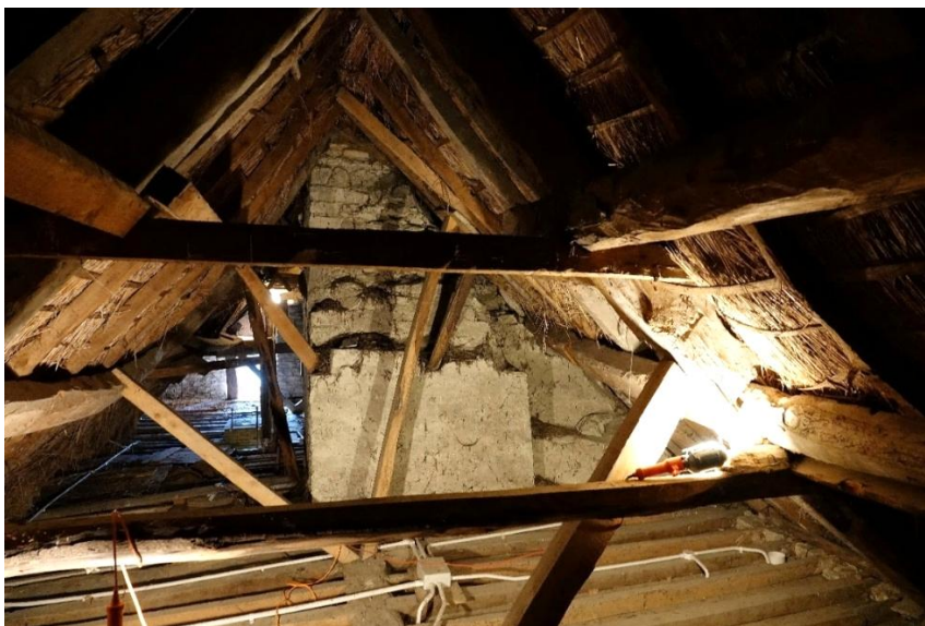
Fig.84 – a view from the NE end wall through T2 to the central stack and south-westwards. The upper purlins and both the collars in the foreground are secondary as are the numerous props
