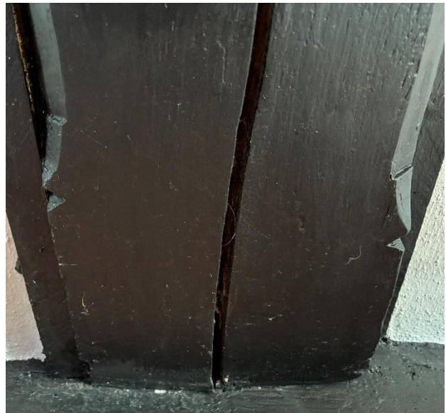
Fig.60 Step and concave stops with nicks, east end of axial beam in bedroom 1
