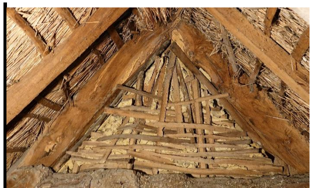
Figs. 75 & 76 – (left) plastered face of the upper part of T1, facing to the central stack; (right) the unplastered face to the end wall
