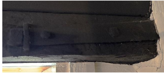
Figs.47 & 48 Straps for wall anchors at south and north ends of west gable end beam
