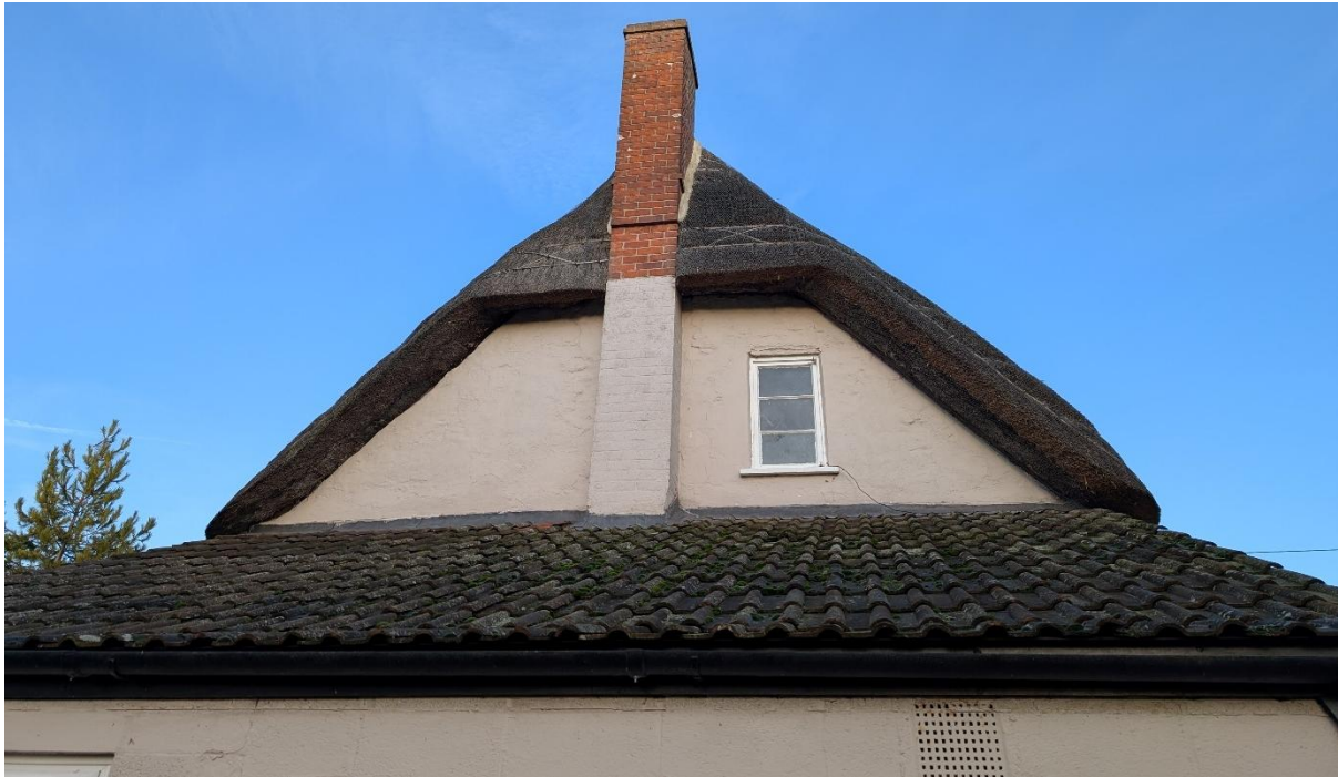
Fig.34c Crittal-type metal-framed window and exterior brick stack
