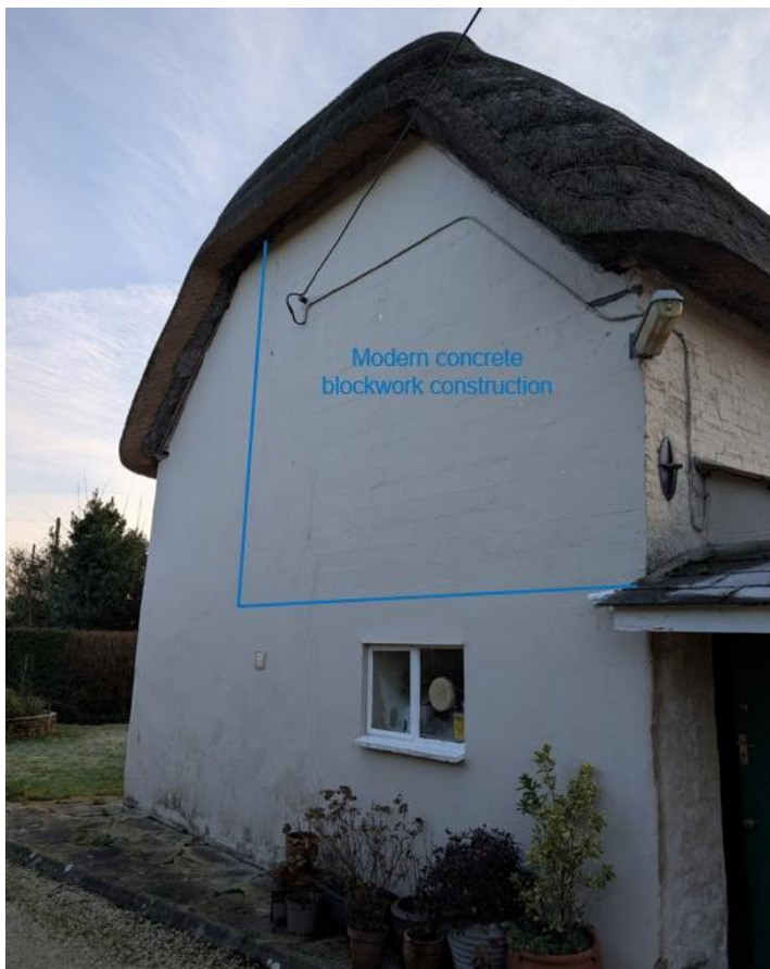
Fig.34b Large area of blockwork refacing on east gable
