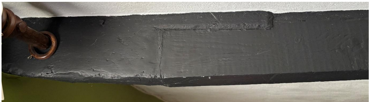
Fig.56 East face of the same beam (above) showing a scarfed-in section of later sawn softwood
