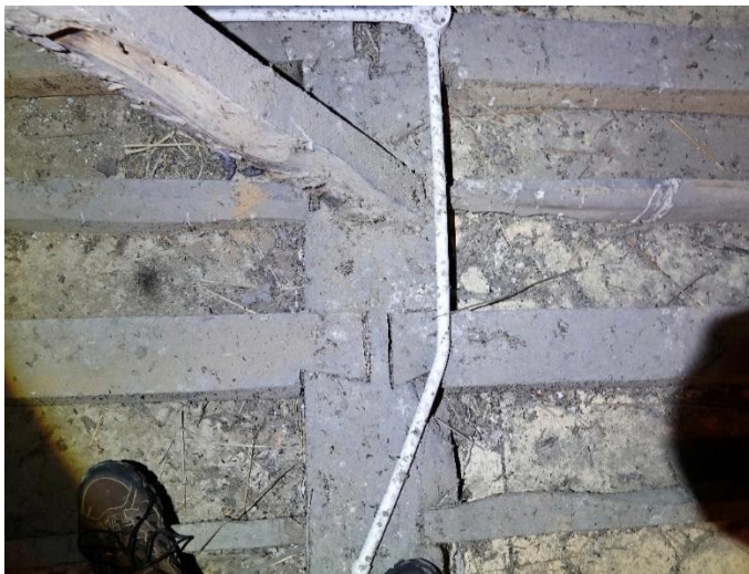
Fig.91 – The spine beam showing the single-dovetail of the heavier joists
