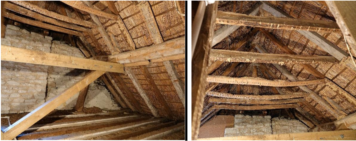
Figs.67 and 68 - (left) the propped purlin in the NW corner of the house (right) lost former ceiling to this bay
