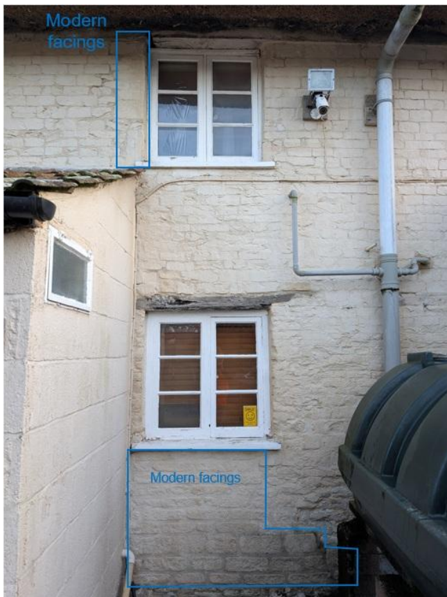
Fig.30 Rear elevation window to east cottage showing replacement facings
