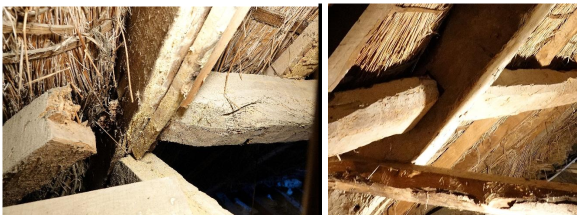
Figs.85 & 86 – details of the purlins showing the butt mortising, and the small cutback - (left) the southern principal of T2; (right) the northern principal of T2, with its single peg just visible
