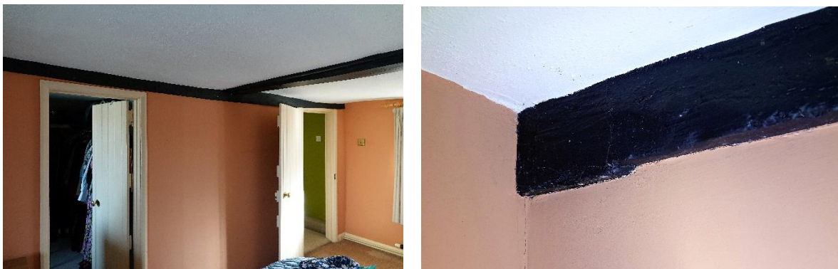
Figs.69 and 70 - (left) the tiebeam of T1, projecting down into the bedroom below, with the spine beam mortised into it; (right) possible remains of a chamfer and stop at the NW end of the tie
