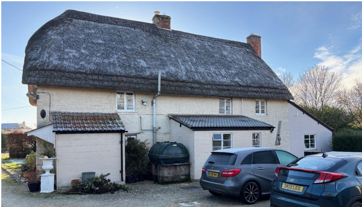
Fig.28 Rear (north) elevation showing the two lean-to entrance porches for nos.2 & 3 Quemerford Gate Cottages, dating from between 1948-1973
