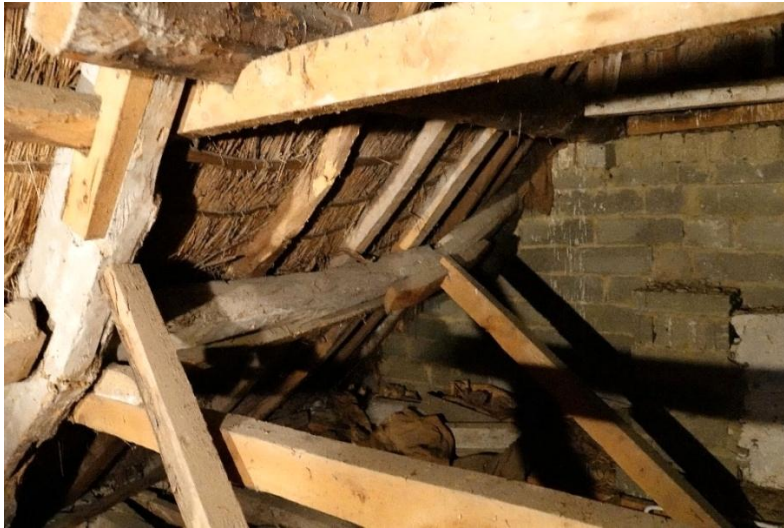
Fig.94 – View along the NW side and purlin of the end bay from T2 in the foreground to the wall
