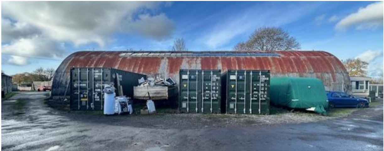
Below: south east elevation of building to be converted:
