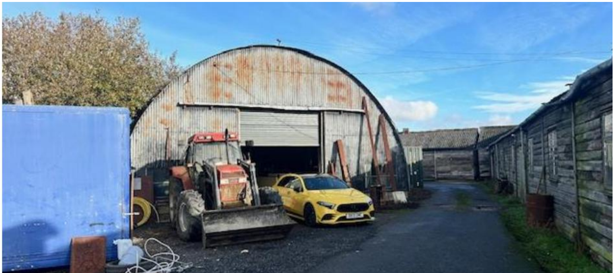
Below: south west elevation of building to be converted:
