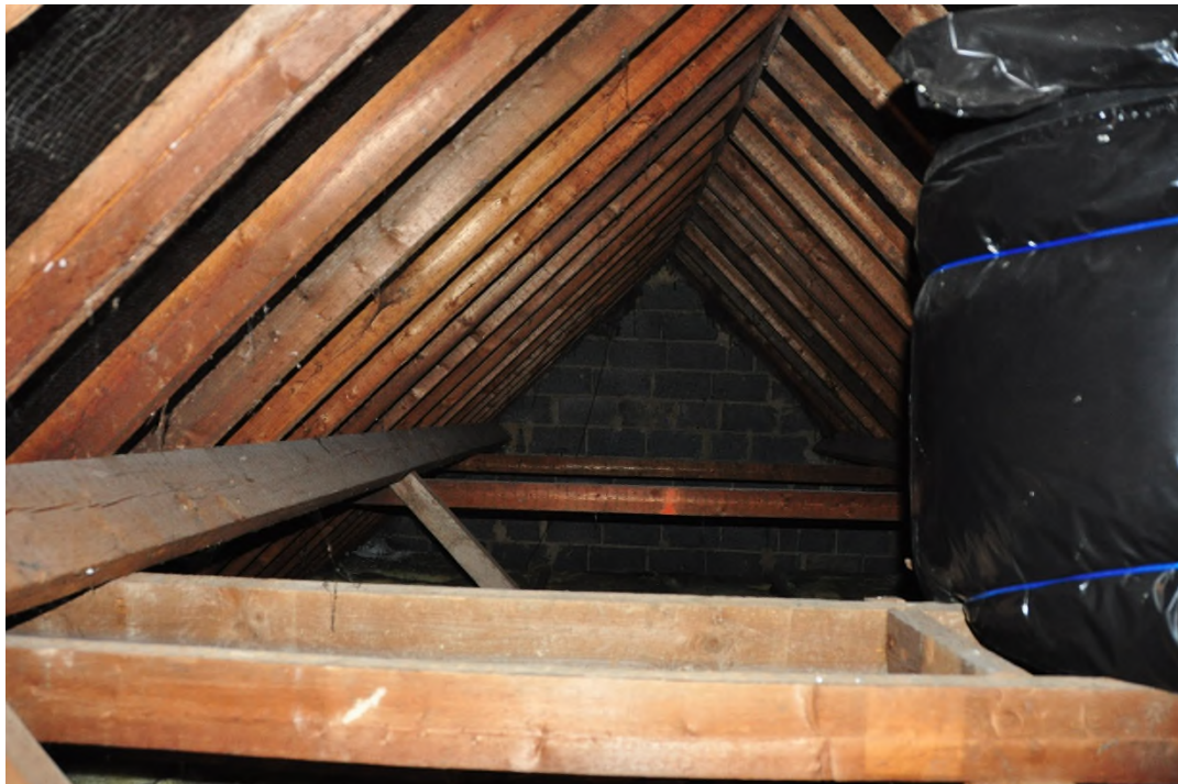
Plate 2 purlin and common rafter construction, no evidence of birds or bats
