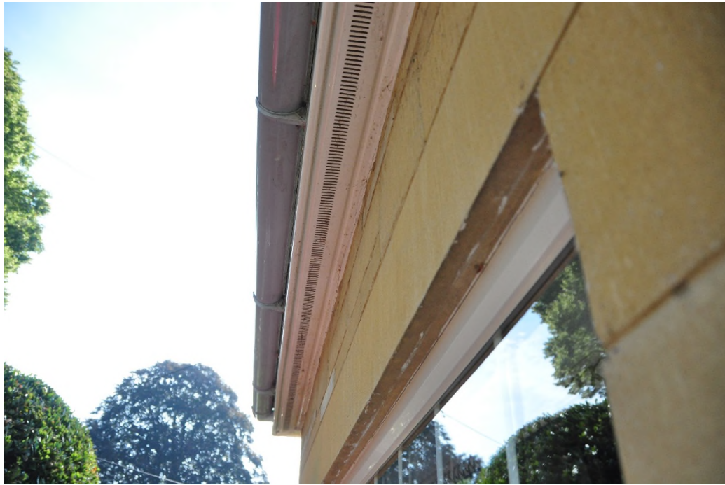
Plate 7 fascia's well sealed and stonework tightly finished no potential for birds or bats
