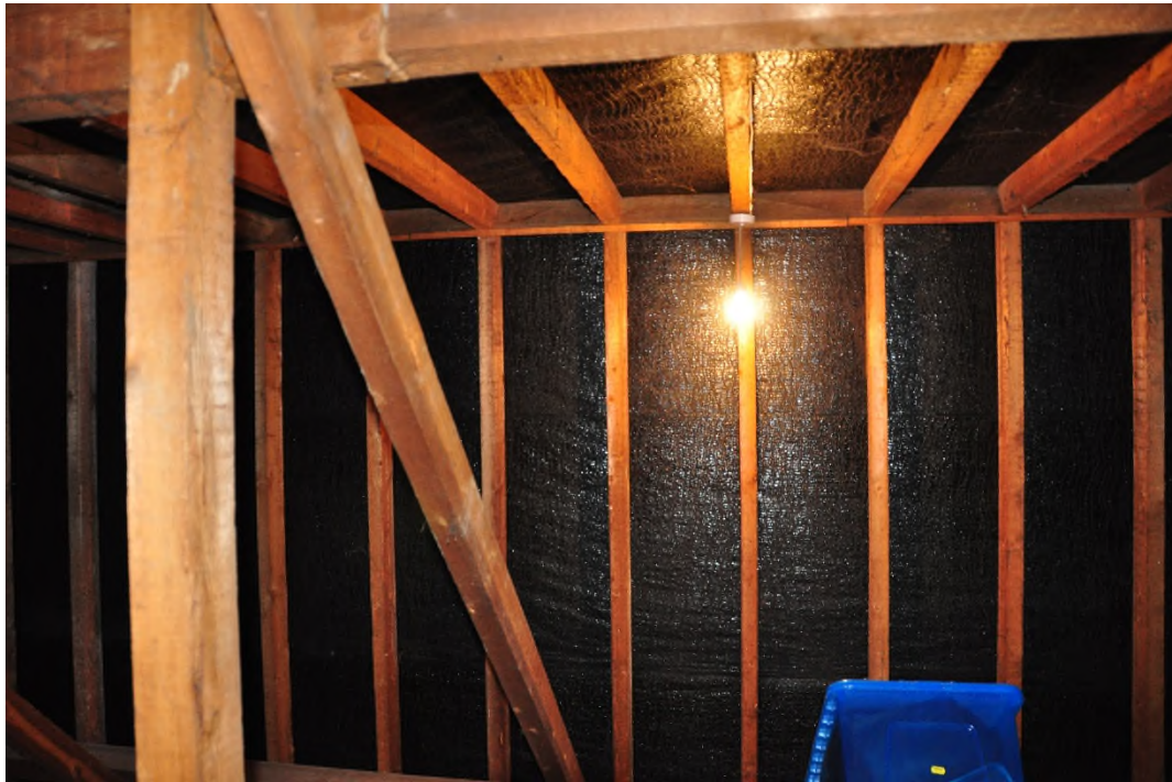
Plate 3 roofing felt in good condition no rips or tears
