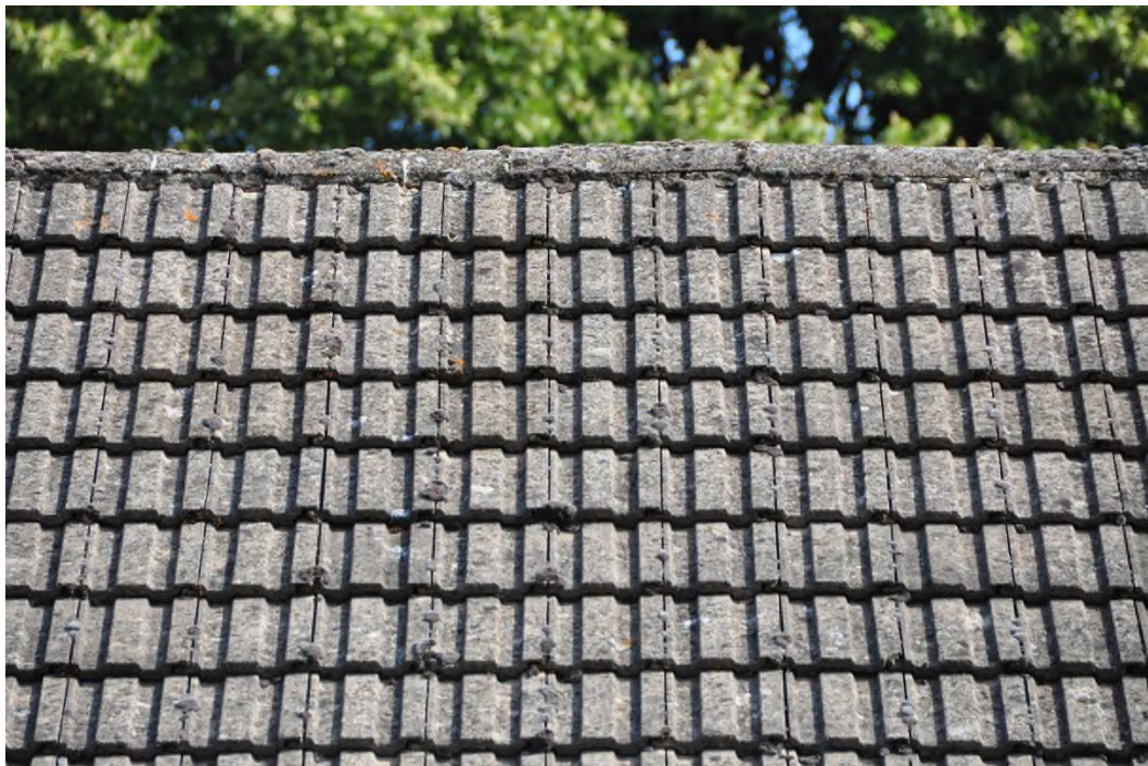
Plate 10 well maintained and finished roof area negligible potential for birds of bats
