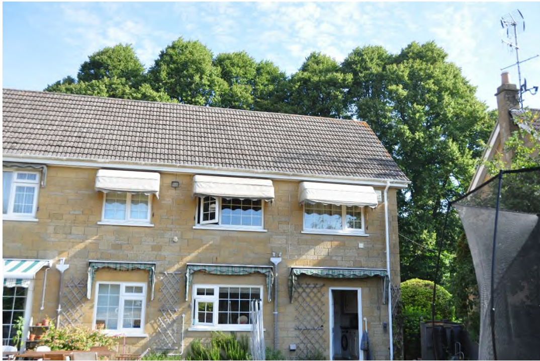
Plate 9 well maintained roof area and tightly finished stone work
