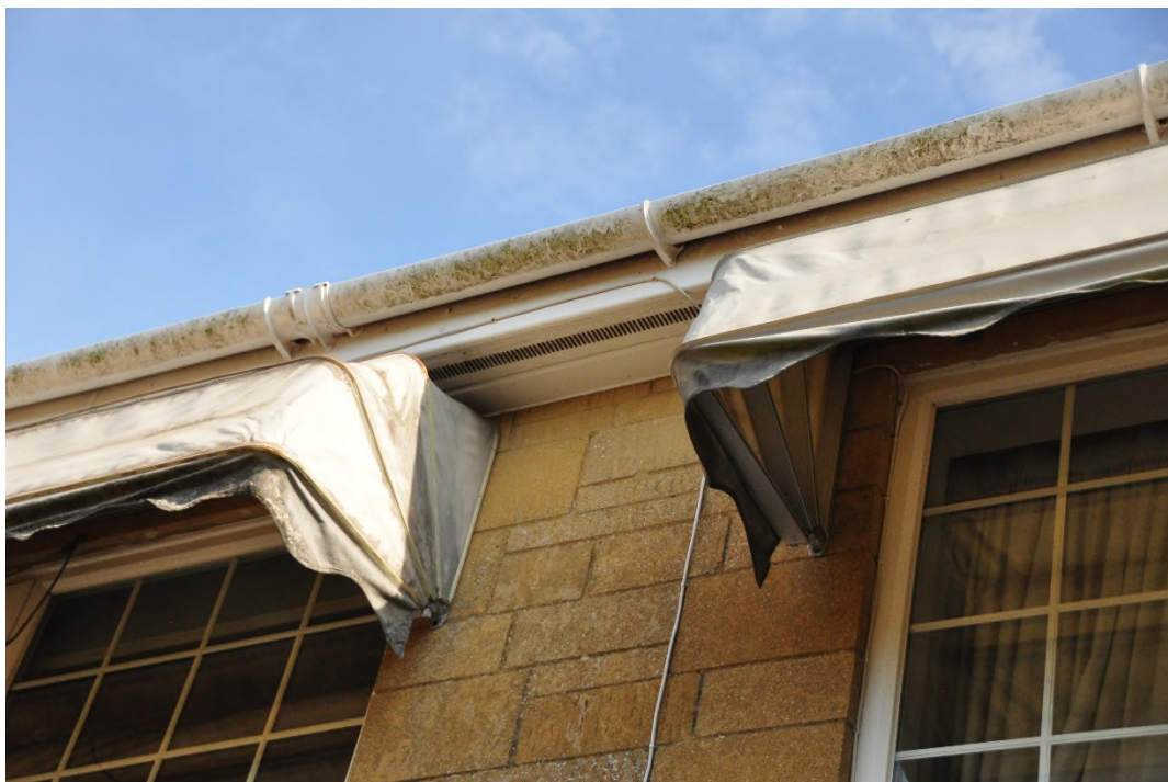
Plate 4 tightly sealed soffit box at the rear of the property
