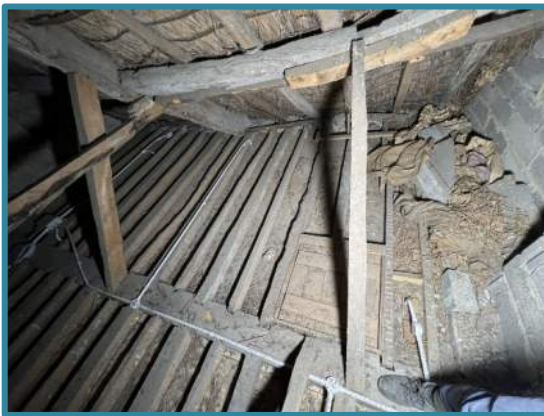
East Cell – Floor Beam
