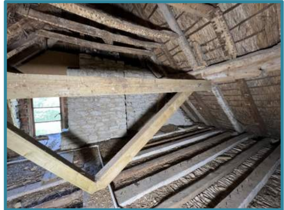
West Cell – Support Frame to Purlins
