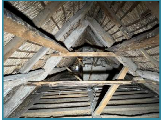
Truss TR1 – Looking West
