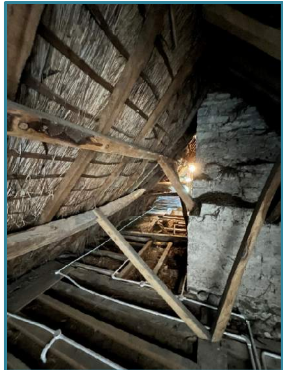
Central Chimney - Looking West
