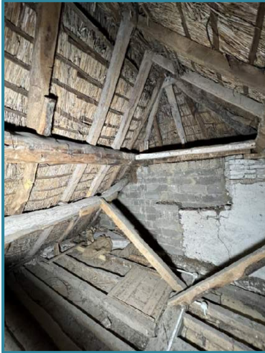
East Cell - Looking East
