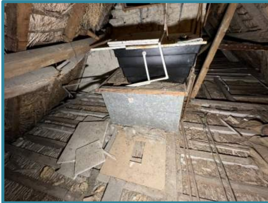
West Cell – Ceiling Structure
