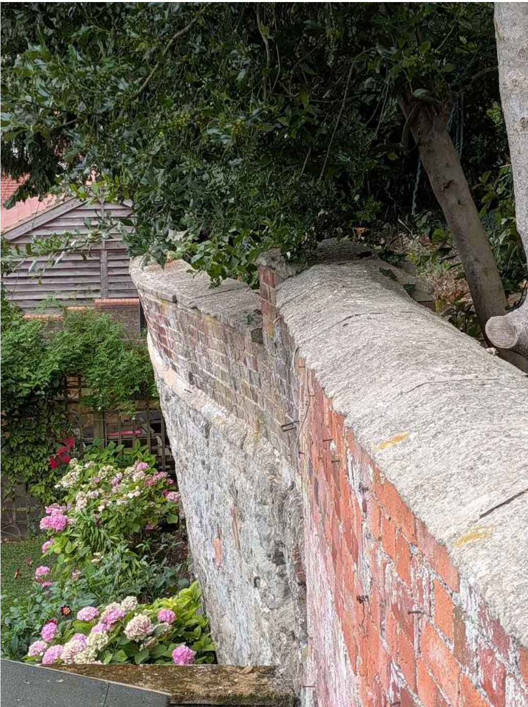
RETAINING WALL VIEWED FROM THE RIGHT
