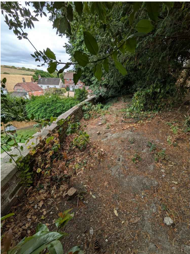
RETAINING WALL VIEWED FROM BRATTON HOUSE
