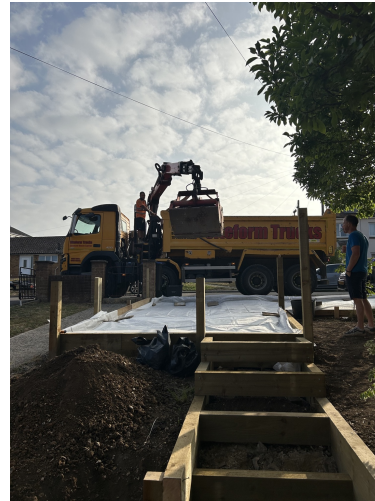
DURING WORKS - geotextile membrane, hardstanding formation, timber retaining work, fence posts and central steps/path.
