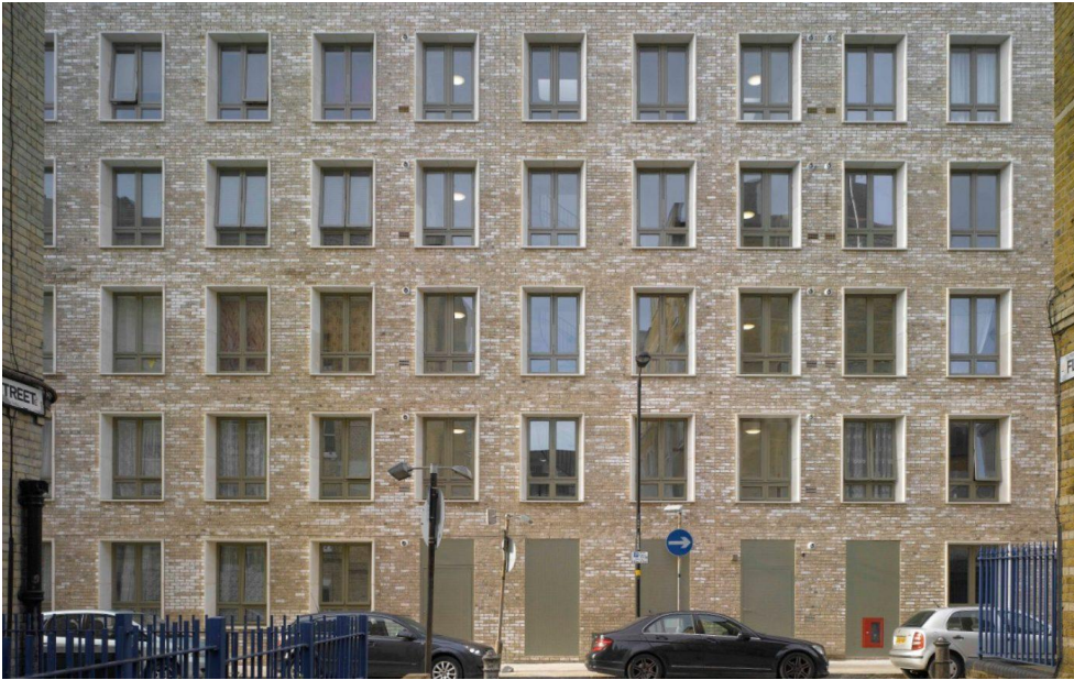
Darbshire House – Niall McLaughlin architects. Here elegant tapered reveals have been used to provide depth, articulation and shadow to the façade.
