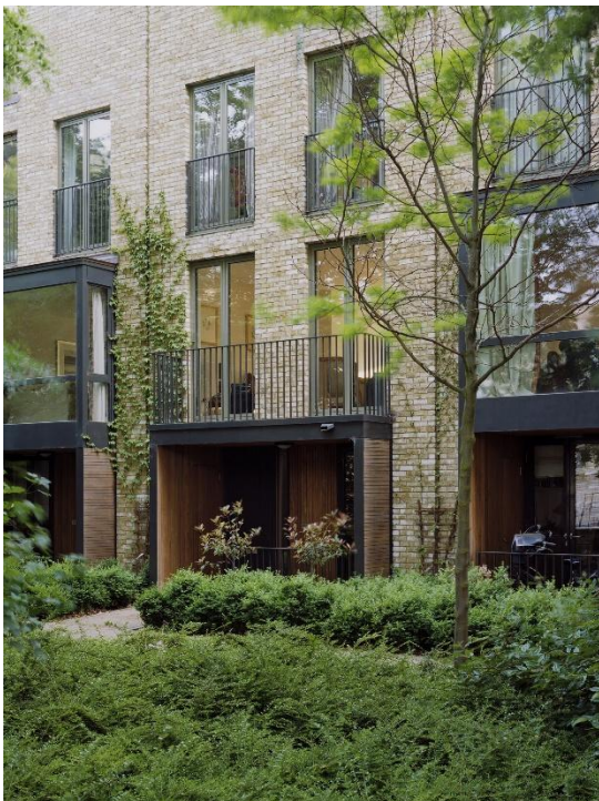
Tall Georgian Window proportions on a contemporary scheme (Maccreanor Lavington Architects, Accordia)
