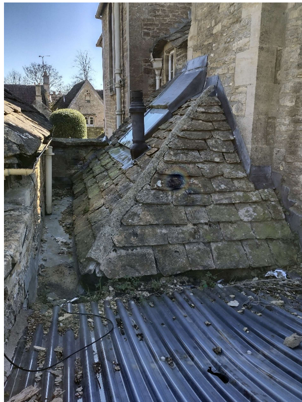
Fig 10: Wood store roof and polycarbonate sheeting
