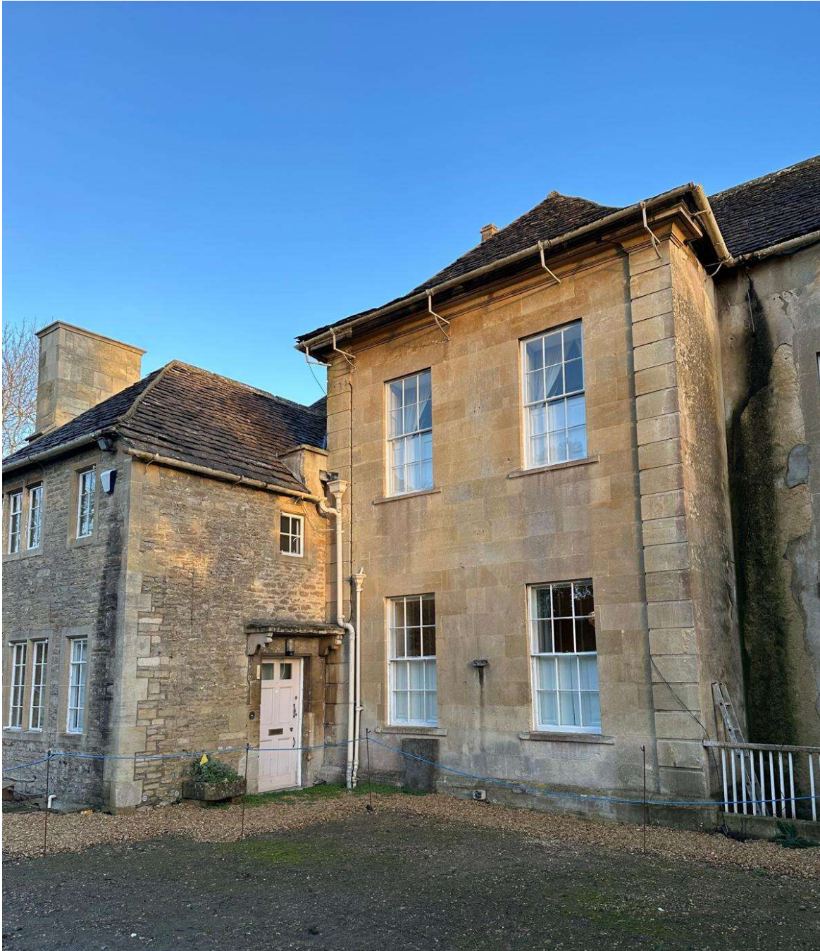
Fig 1 Rubble façade to be lime rendered, adjacent ashlar dressed façade on the right.
