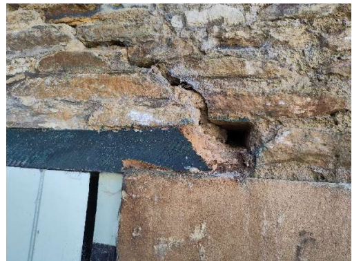
Fig 5: (top) wood store west façade Fig 6: (above) rotten wood lintel Fig 7: (left) wood store north facade
