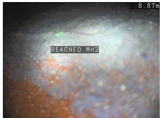
MH1X_769edb1c-839f-4c4d-9e71-f085b70d640a_20241106_123002_979.jpg, 00:02:43, 8.87 m Finish node, manhole, reference: MH2
