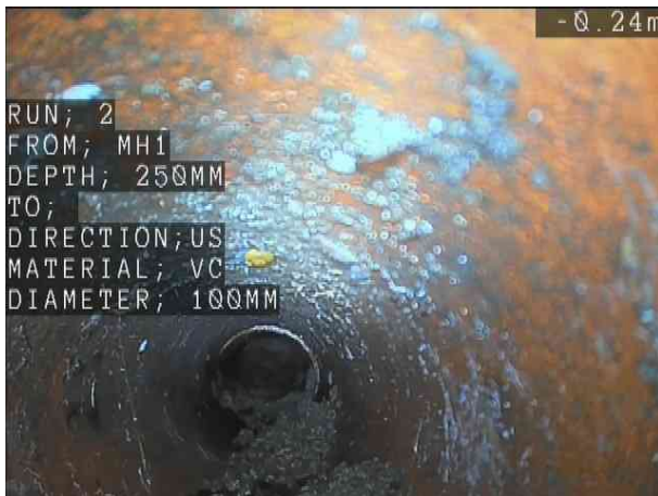
UnknownX_279483a8-278f-4339-bbc0-710ba6033481_20241106_122259_767.jpg, 00:00:00, 0.00 m Start node, manhole, reference: MH1
