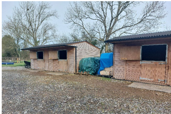
View looking northeast at the existing mobile stables.
