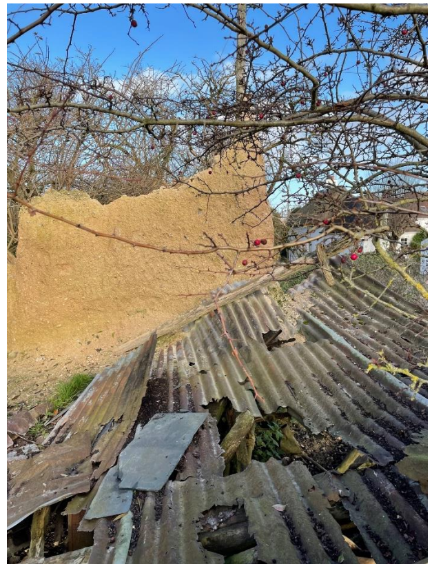
SOUTH WEST ELEVATION – Evidence of corrugated roof structure adjacent cob barn
