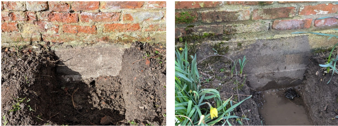
Figure 8 trial pit at rear (no underpinning) and trial pit alongside (underpinning present)
