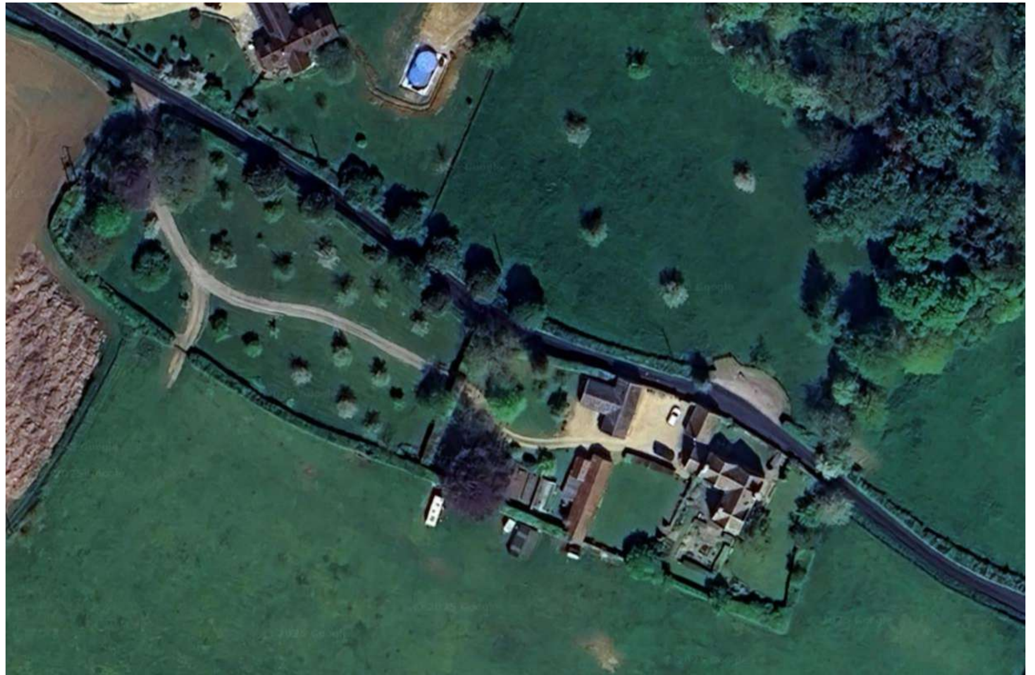
Aerial view of Coles Farm, Google Maps, 2025
