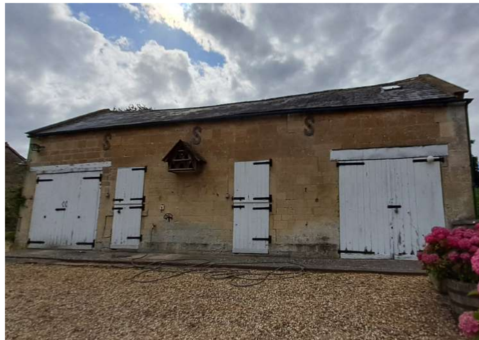
South-East elevation of the Stable
