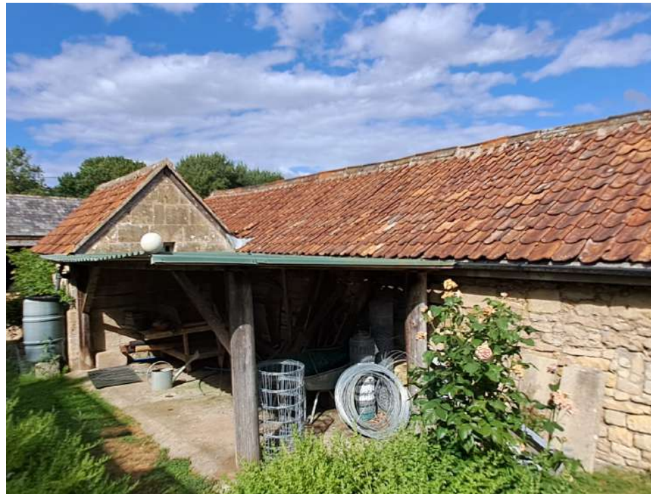
North-West elevation of the Cowshed
