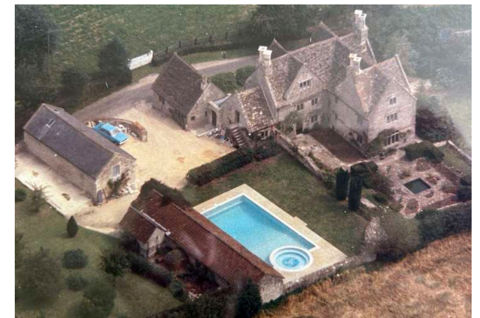
A 1970s aerial photograph showing the house after the works by Lady Juliet de Chair, including the creation of new swimming pool and the conversion of the neighbouring Cow Shed into a pool building.
