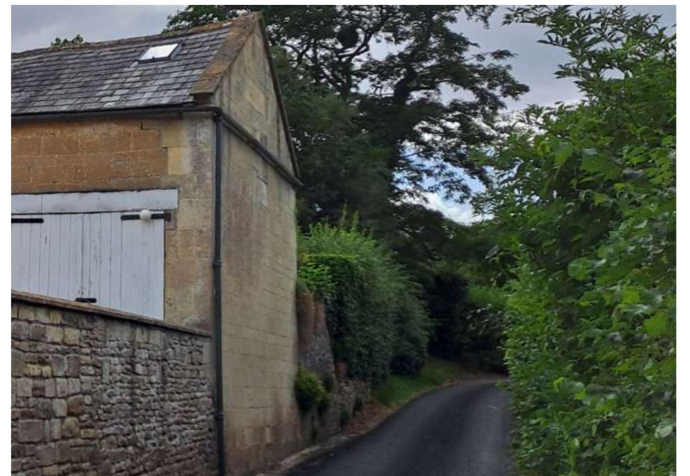
North-East elevation of the Stable
