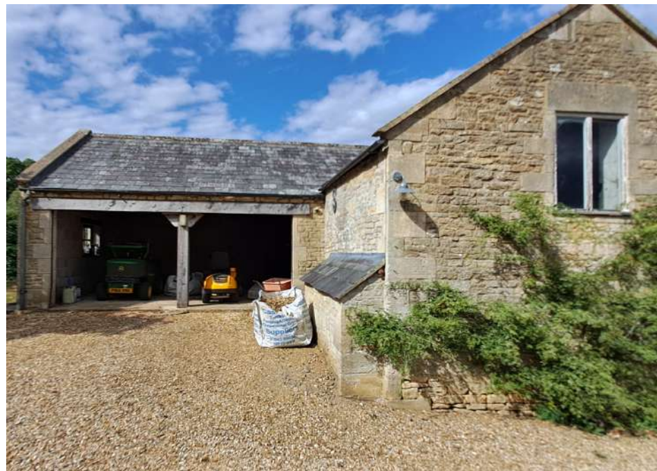
South-West elevation of the Stable
