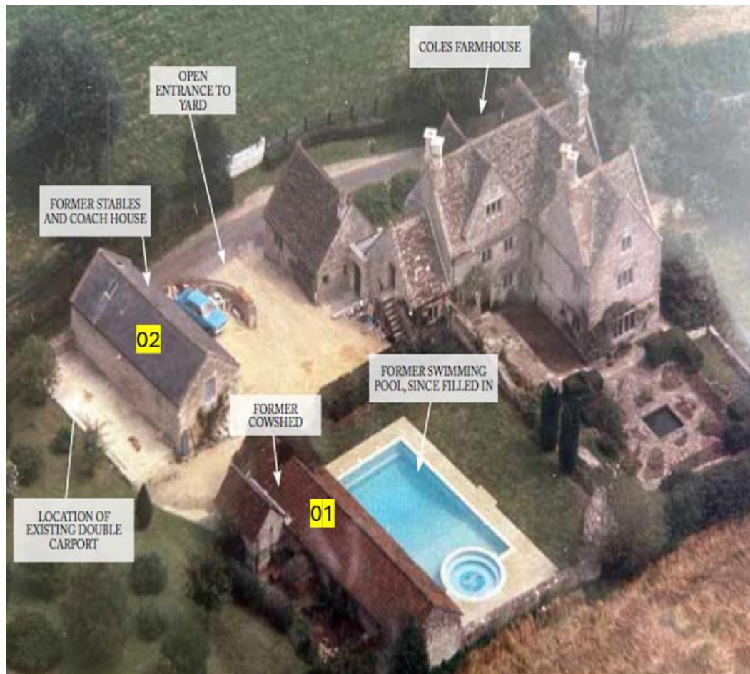
Figure 1 Aerial view of c.1973 showing the works in progress and the creation of the new swimming pool
