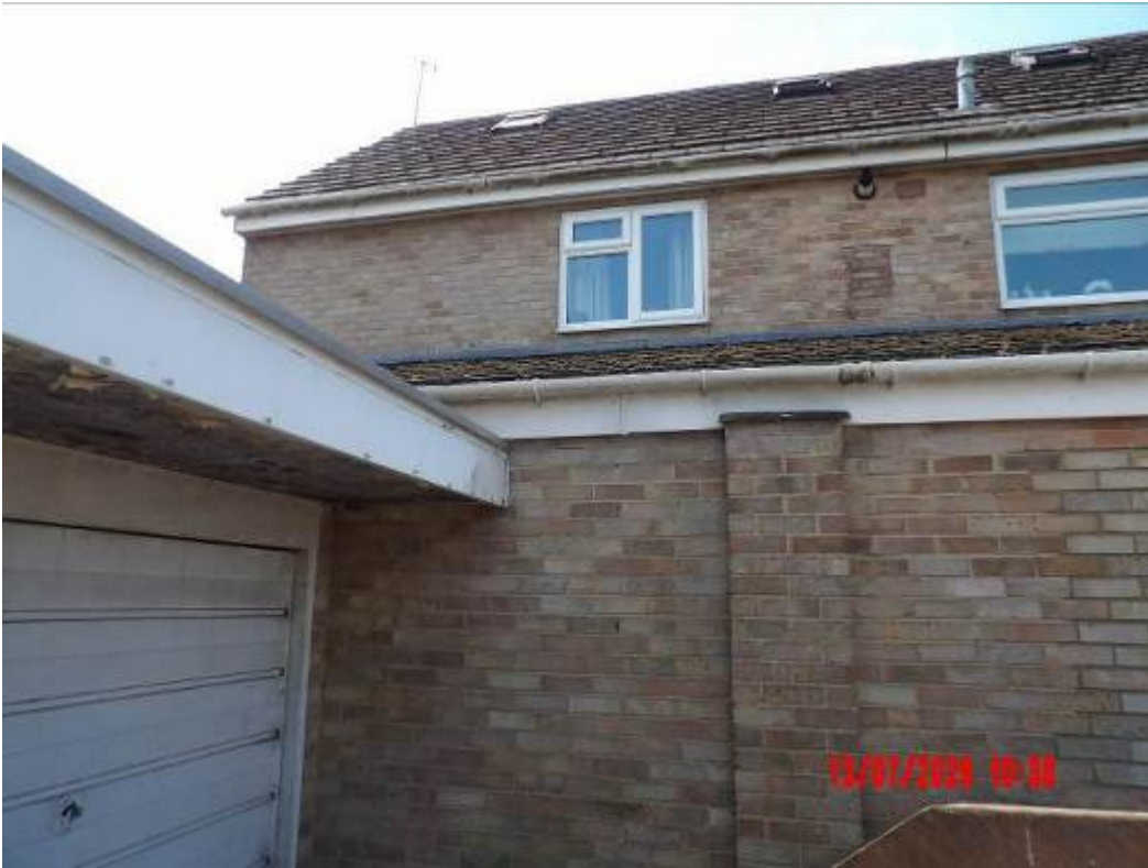
1. PARTIAL FRONT ELEVATION SHOWING NEIGHBOURS GARAGE.
