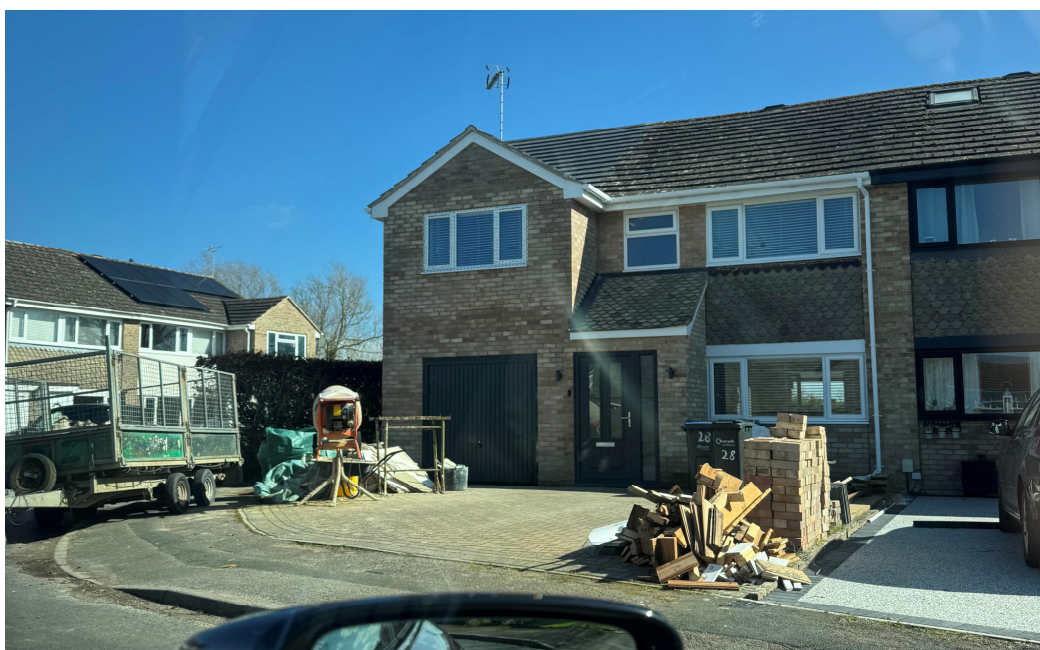
16. No 28 - Gable Fronted Extension (Real-time Photo).
