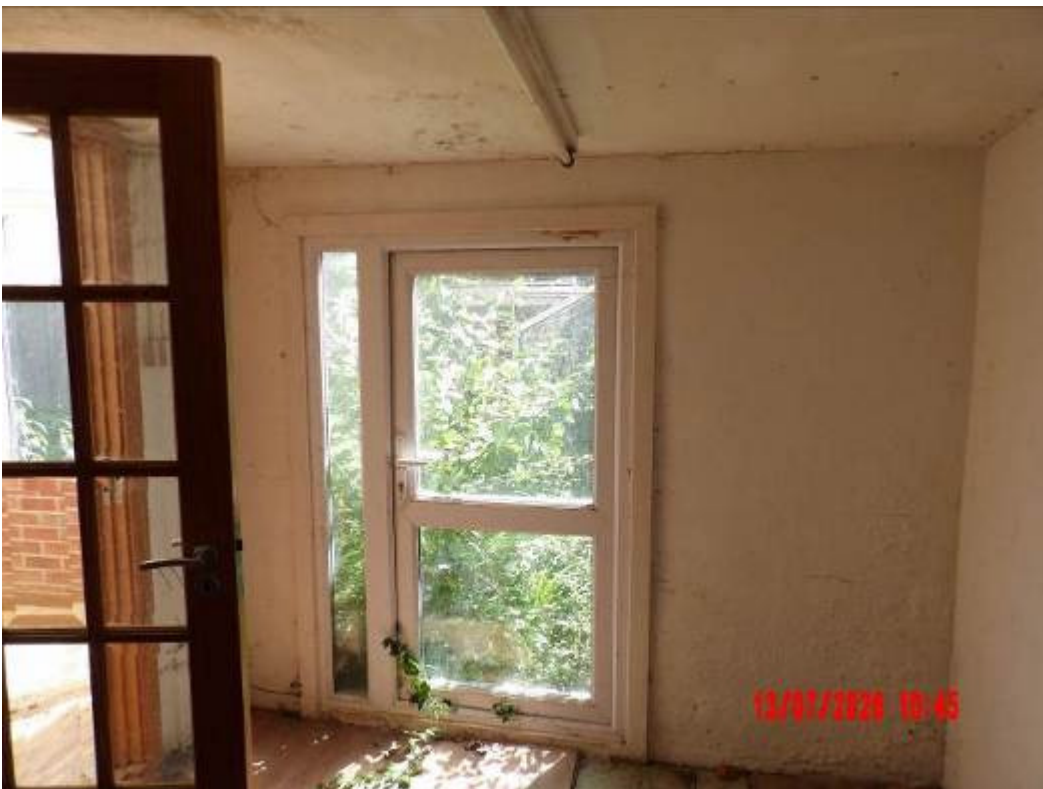
12. WORKSHOP TO REAR OF GARAGE.
