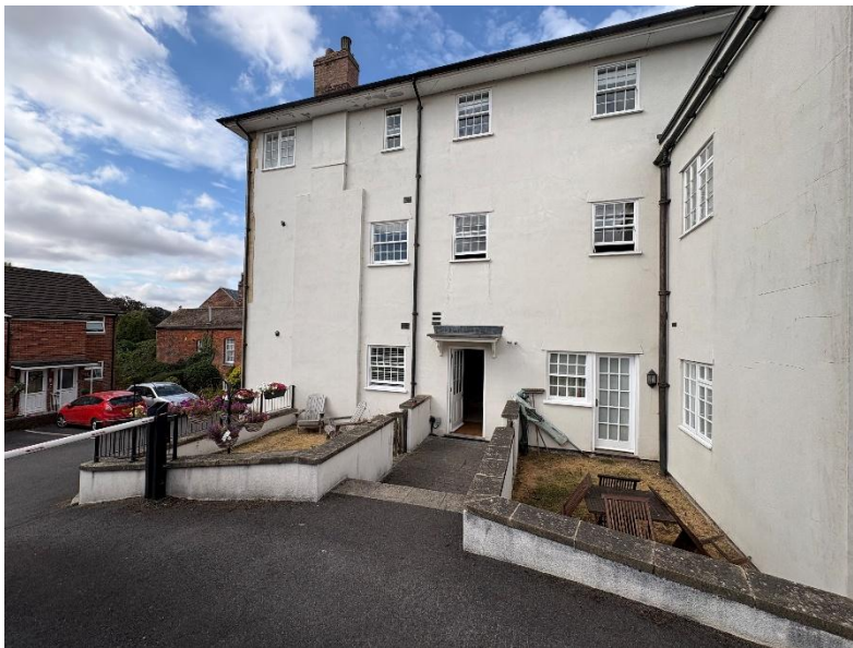
Figure 1 - Silbury House - Rear Elevation
