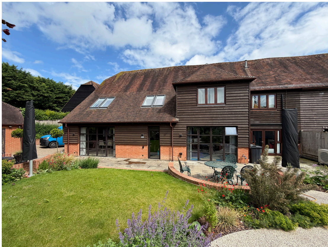
Image 1 The existing rear elevation of Mulberry Barn.
